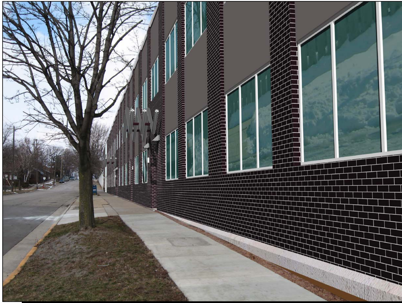
WEST ELEVATION OF NORTH DICKINSON STREET - SIDEWALK
