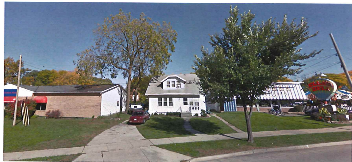
7 EXISTING CONDITIONS - VIEW NORTH
