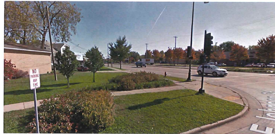
4 EXISTING CONDITIONS - VIEW SE
