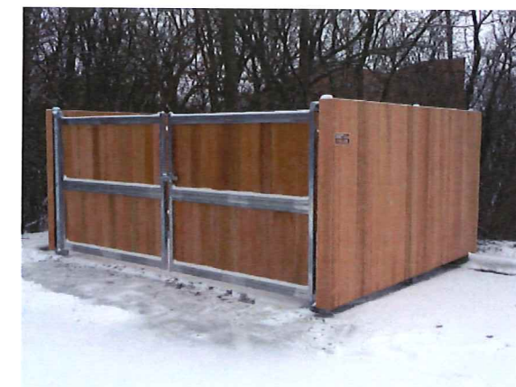
3 DUMPSTER ENCLOSURE 6' HIGH C102 NTS
