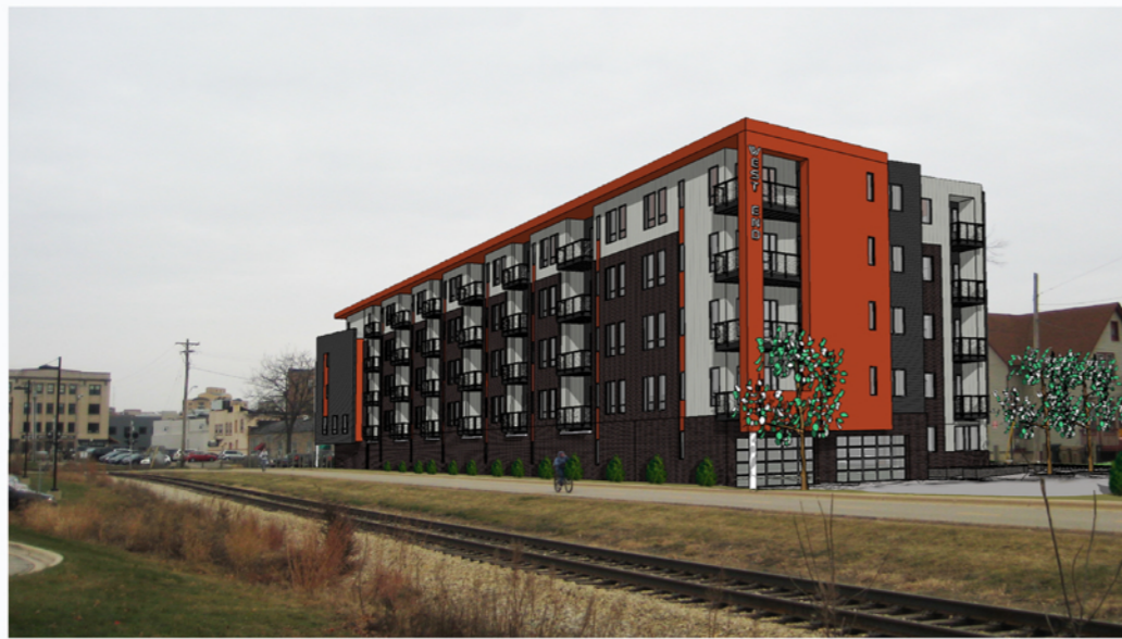
View From South Along Bike Path
