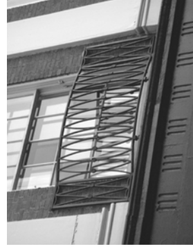
2 Painted Metal Railing Reference Image SCALE: N.T.S.
