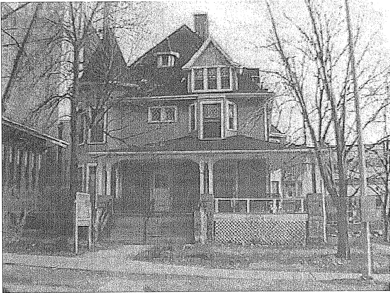
309 N. Mills Street proposed for demolition for multi-story apartment building see attached
