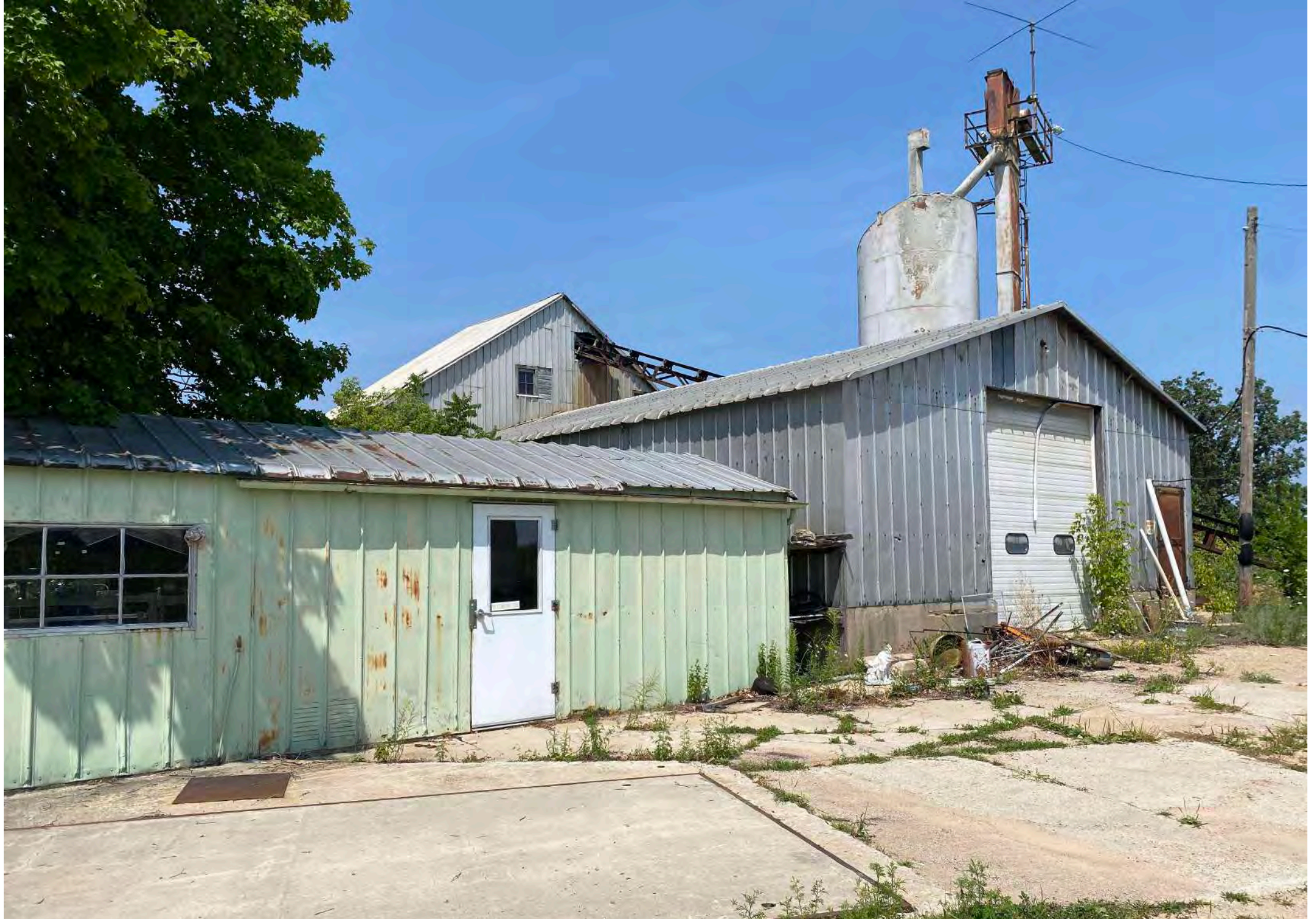
3450 Milwaukee St. - Office Outbuilding
