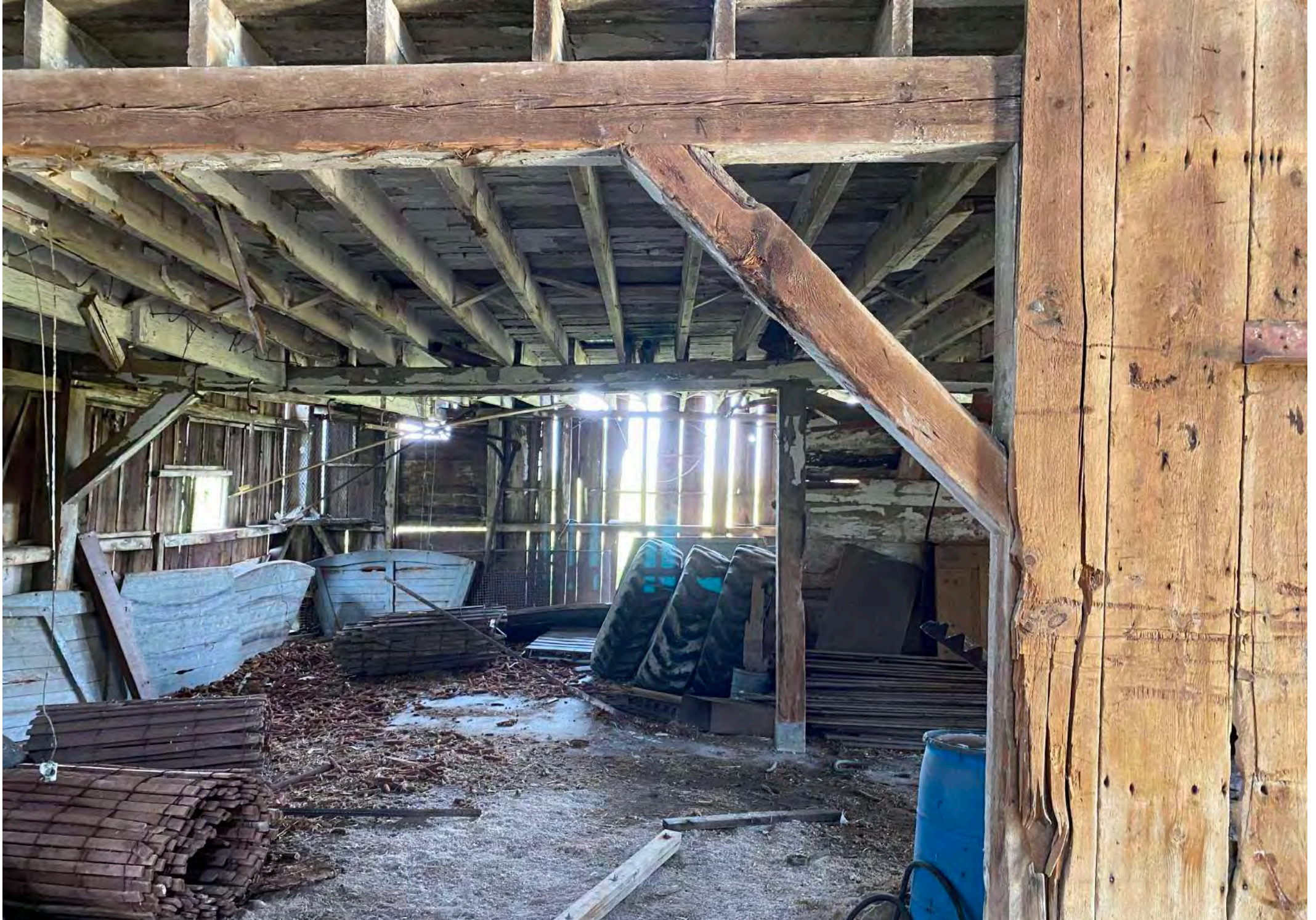
3450 Milwaukee St. - Wood Barn
