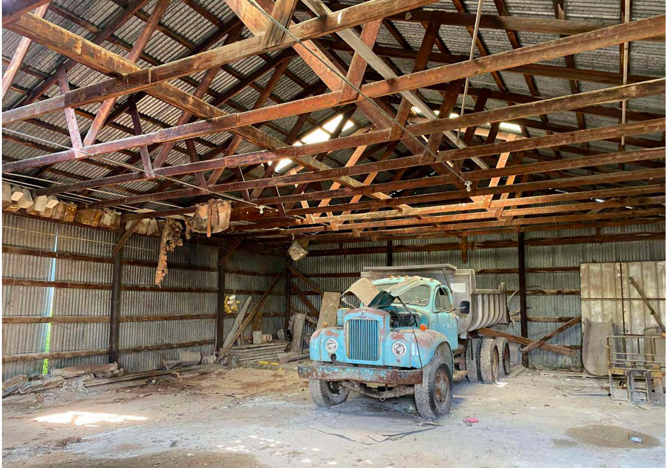
3450 Milwaukee St. - Storage Shed
