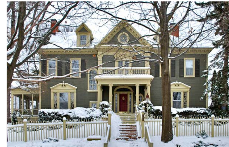
B: 205 N PROSPECT AVE (adjacent to proposed home) roof: hip (shallow overhang) facade: horizontal wood siding
