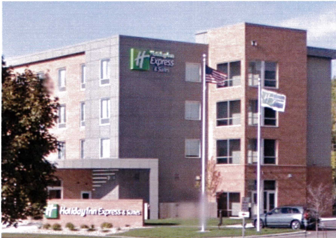
Holiday Inn Existing Wall Sign (3) – East Elevation Sign is 66 Square Feet
