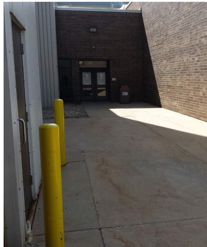
SOUTHWEST CORNER OF LOADING DOCK
