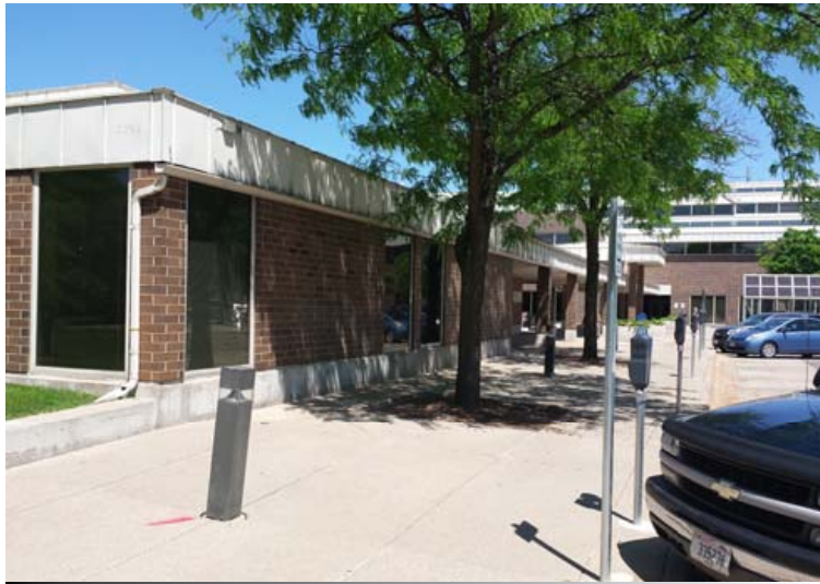
ADMINISTRATIVE BUILDING - EAST FACE
