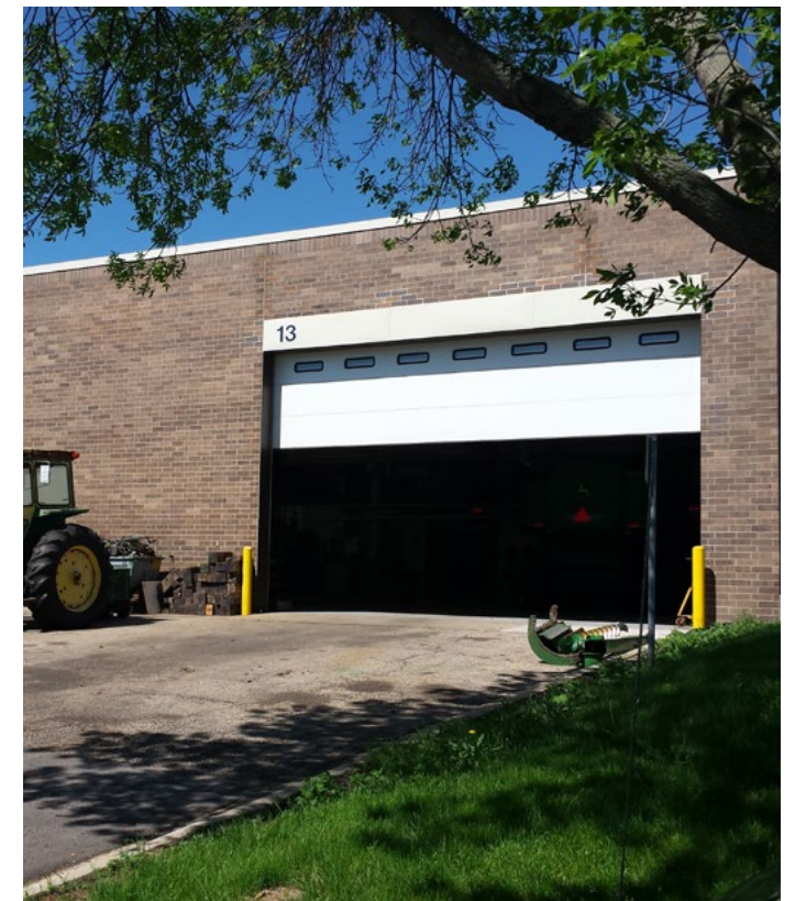
VIEW SOUTHWEST FROM ENTRY DRIVE
