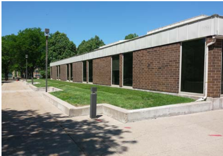
ADMINISTRATIVE BUILDING - SOUTH FACE
