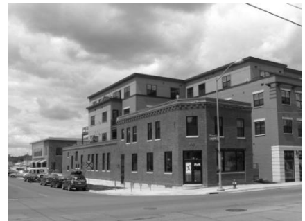
B1. Facade articulation
