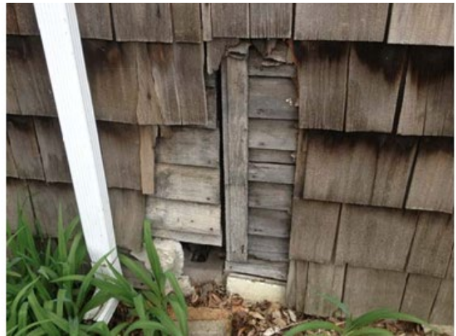
2014 Photos showing historic clapboard under shingle siding
