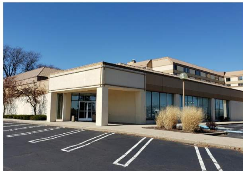
4402 East Washing ton Avenue – Exterior No. 5
