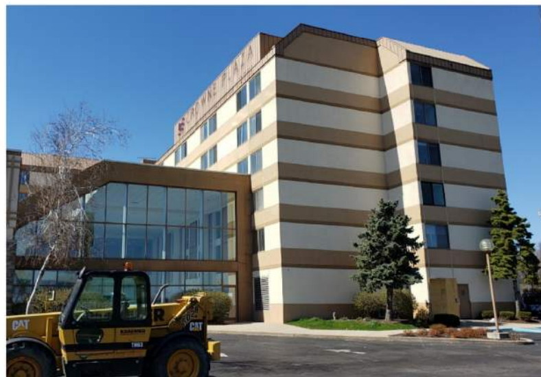
4402 East Washing ton Avenue – Exterior No. 6
