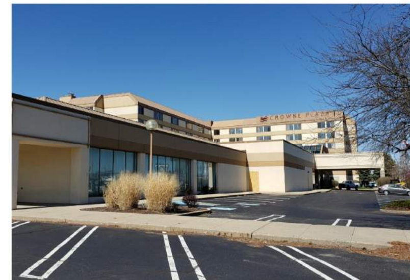
4402 East Washing ton Avenue – Exterior No. 4
