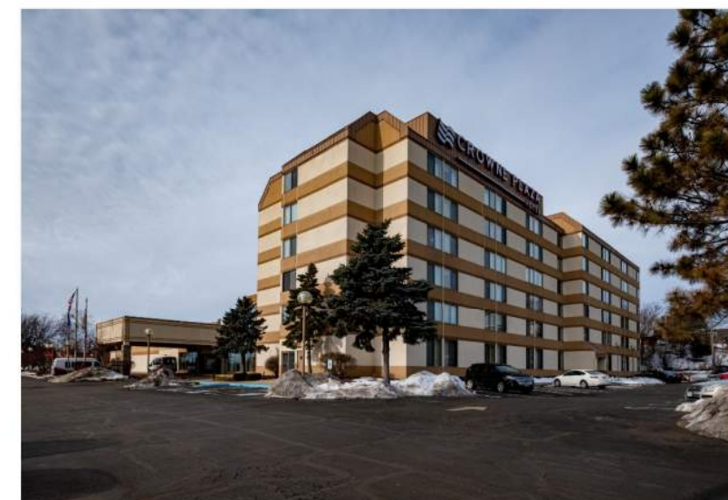
4402 East Washing ton Avenue – Exterior No. 1
