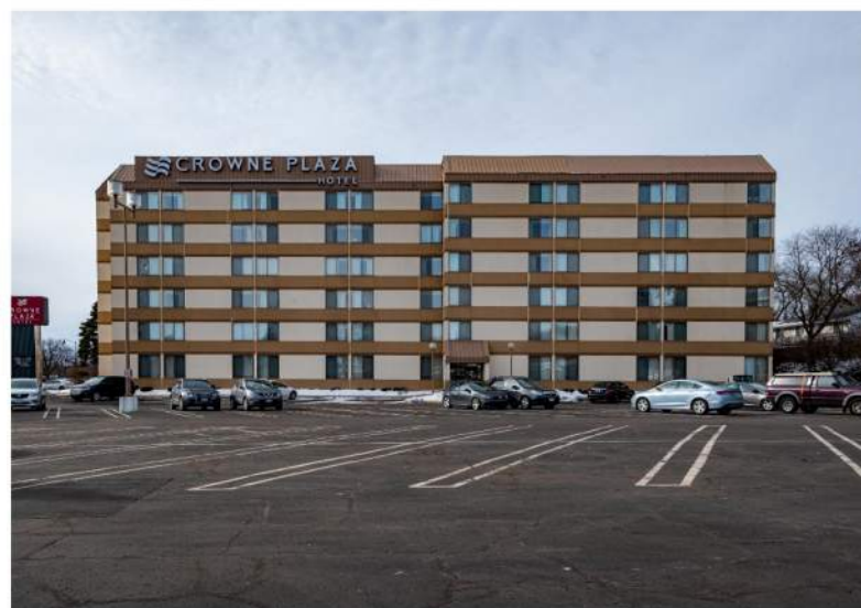
4402 East Washing ton Avenue – Exterior No. 2
