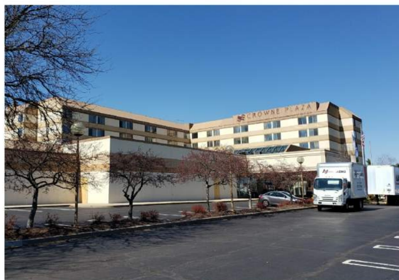
4402 East Washing ton Avenue – Exterior No. 3
