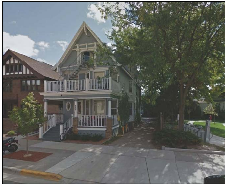
EXISTING BUILDING AND PARK ON GILMAN
