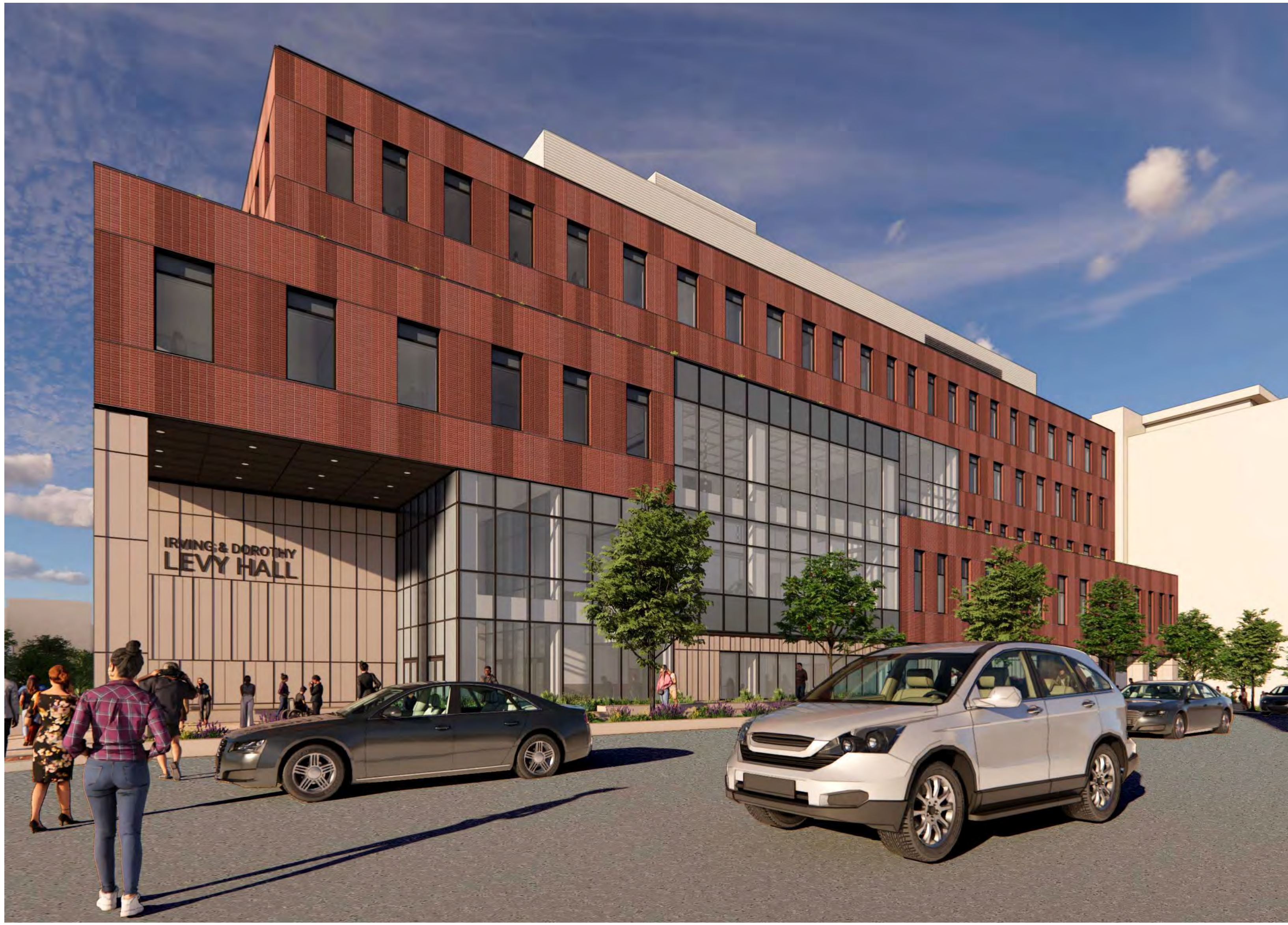
Overall - North Facade
