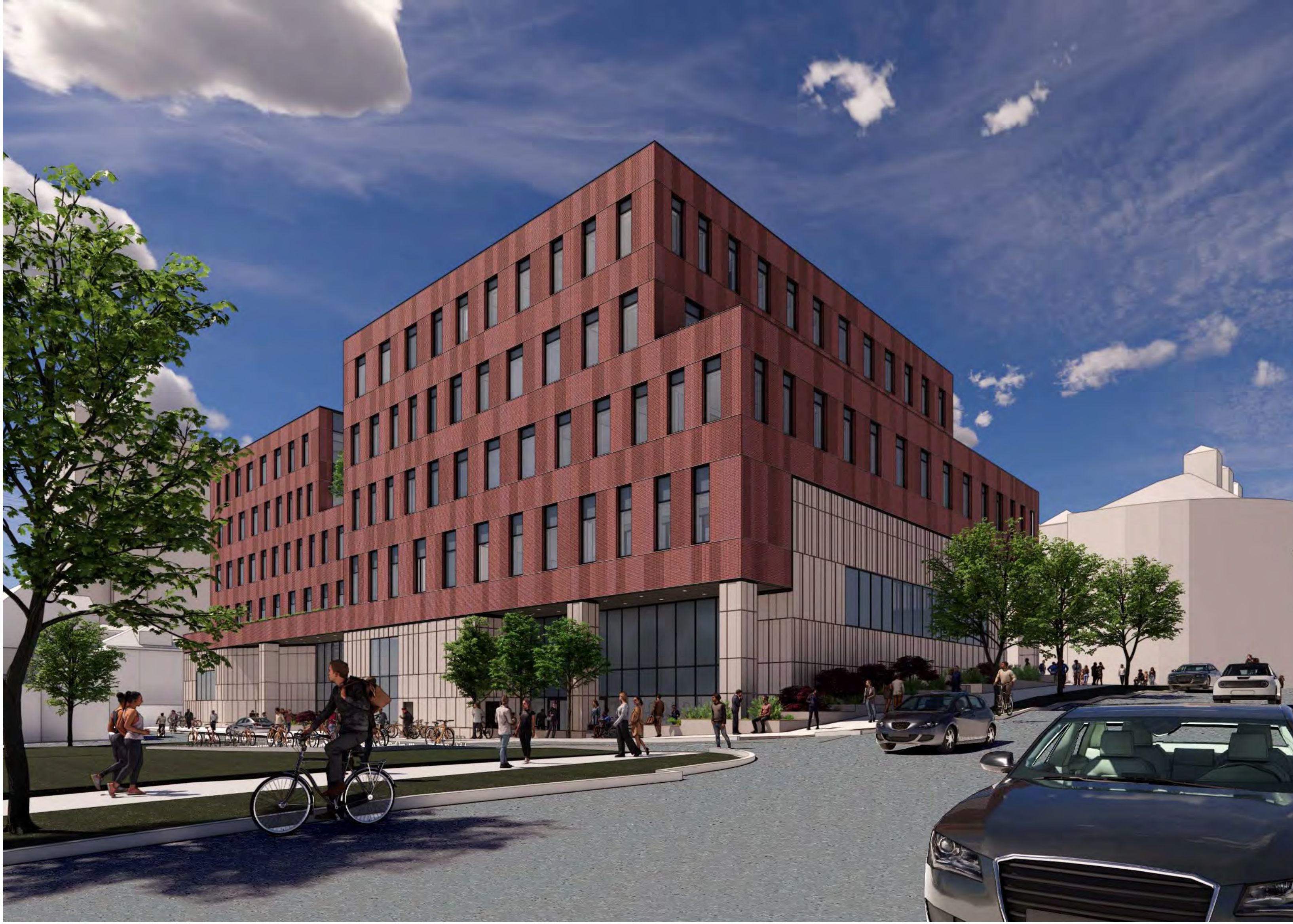
Overall - Park Street - Looking North
