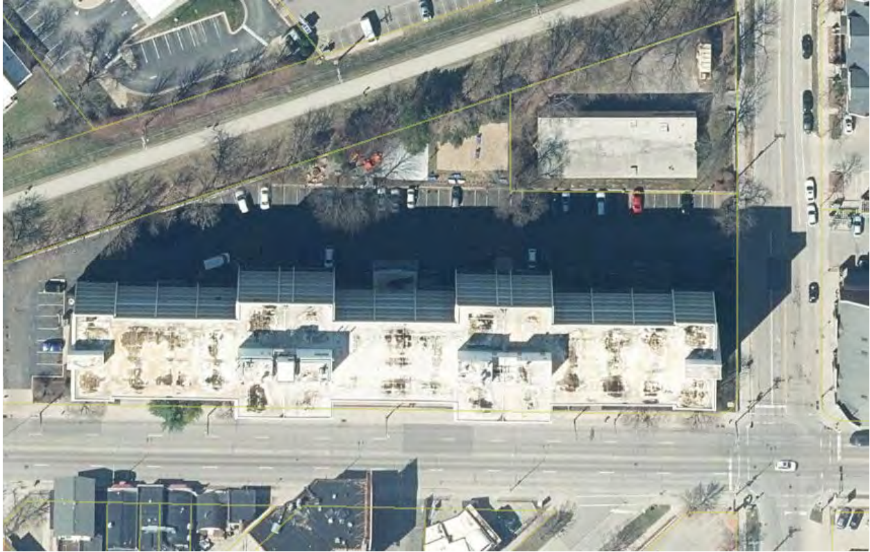
1402 Regent Street – The Regent Apartments (approximately 19' front setback)
