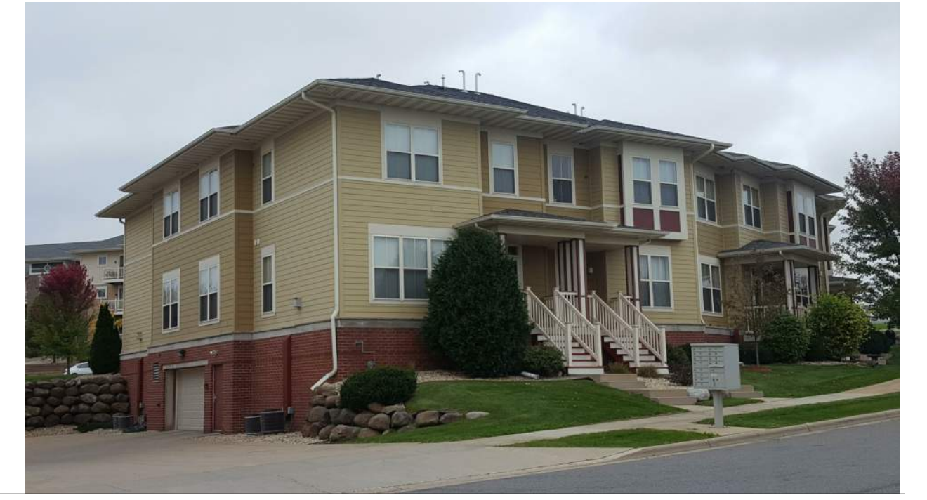
View from Felland Rd. to S.E. Corner of 9 Unit Bldg.
