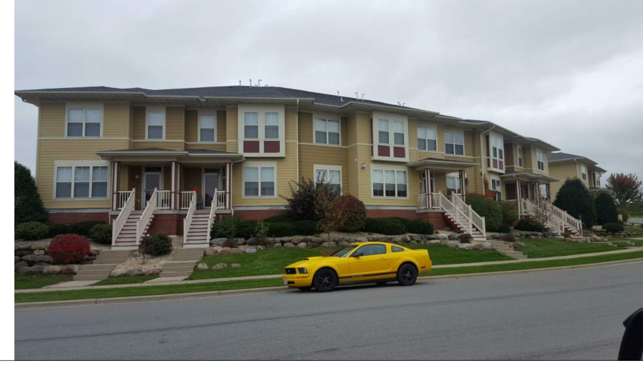
View from Felland Rd. to S.E. Corner of 9 Unit Bldg.
