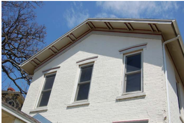
Detail showing triangular stone pediments and paired modillions.
