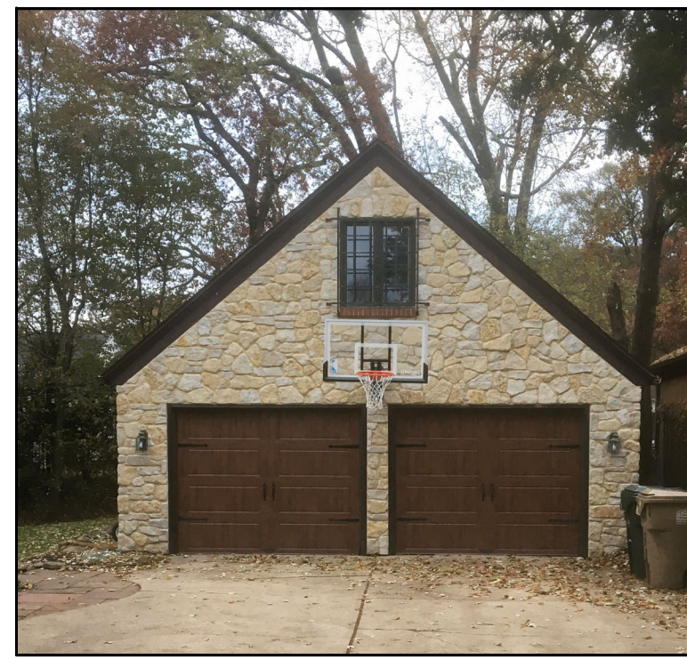
Existing Garage Front (East) Elevation
