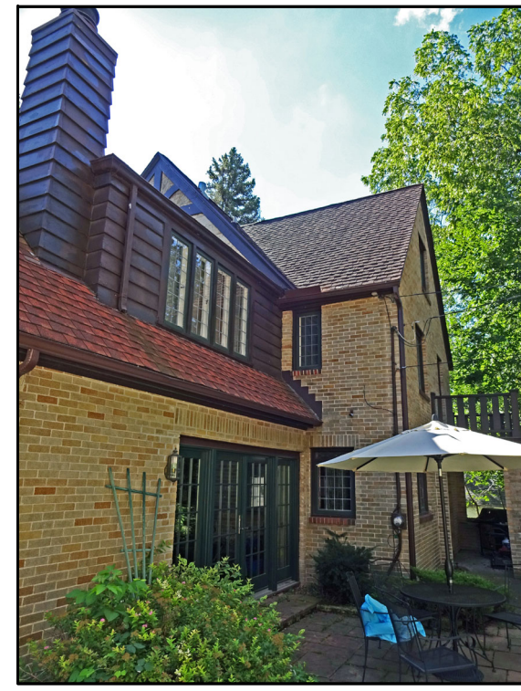
Existing House Back Yard (West) Elevation (sharing back yard with ADU primary south elevation)
