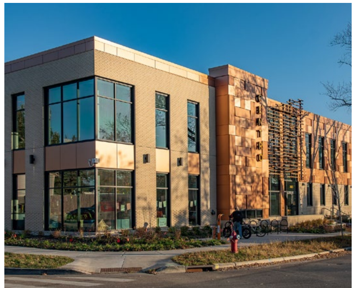
The new Centro Hispano facility on Cypress Way
