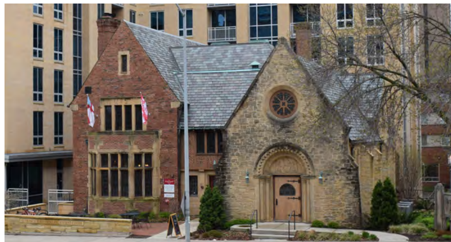
ABOVE: St. Francis House Episcopal Student Center, 1011 University Avenue. The St. Francis House Episcopal Student Center was the site of the first group to organize and publicly advocate for LGBTQ civil rights in Wisconsin in 1969 and the home of many of Madison's leading LGBTQ organizations during the 1970s and 1980s.
