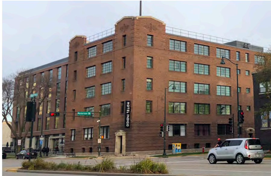
Klueter Wholesale Grocery Warehouse, 901 East Washington Avenue
