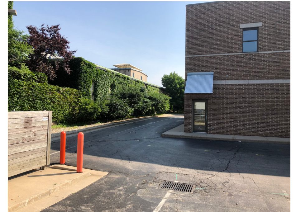
View of Site from West Corner, looking Northeast.
