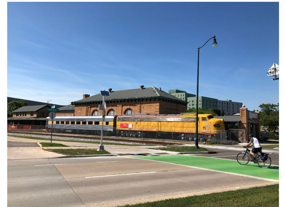
View of building and bike path directly Southwest of Site.
