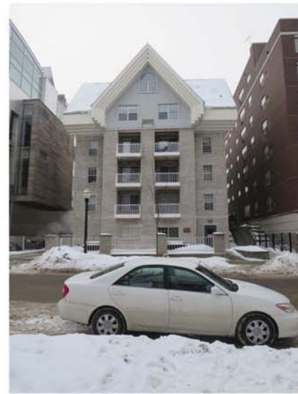
LOOKING ACROSS THE STREET AT 619 LANGDON STREET
