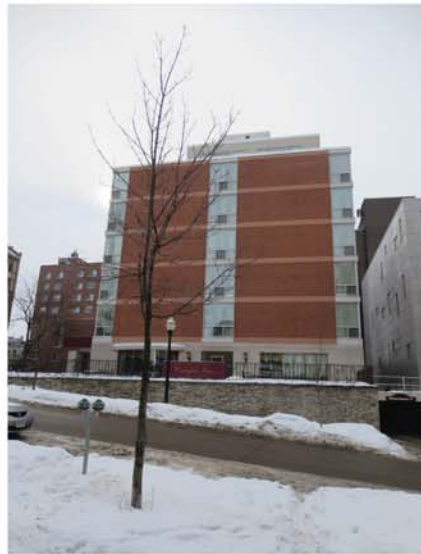
LOOKING ACROSS THE STREET AT 601 LANGDON STREET
