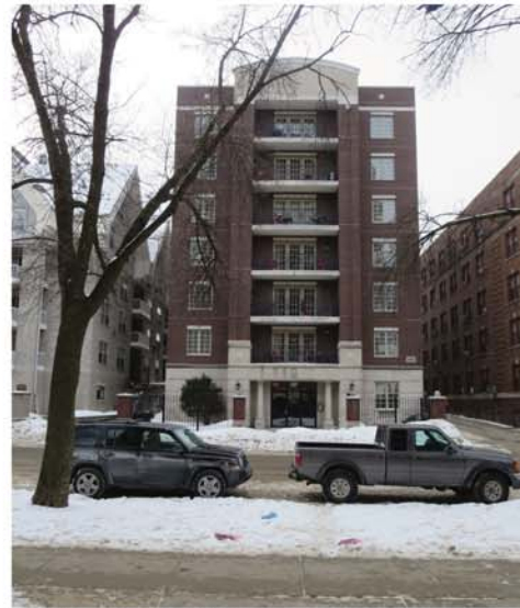
LOOKING ACROSS THE STREET AT 625 LANGDON STREET
