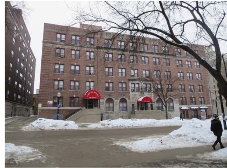
LOOKING ACROSS THE STREET AT 633 LANGDON STREET
