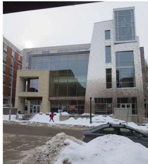
LOOKING ACROSS THE STREET AT 611 LANGDON STREET
