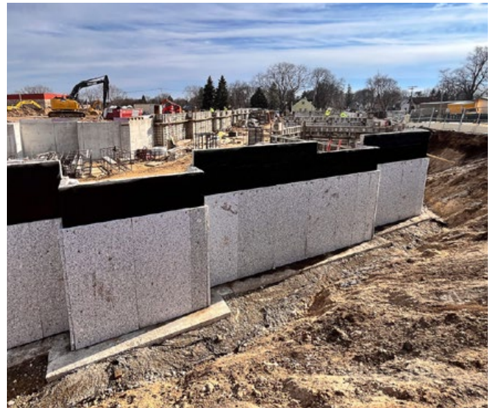
RISE Madison under construction at the former Gardner Baking site on East Washington Avenue
