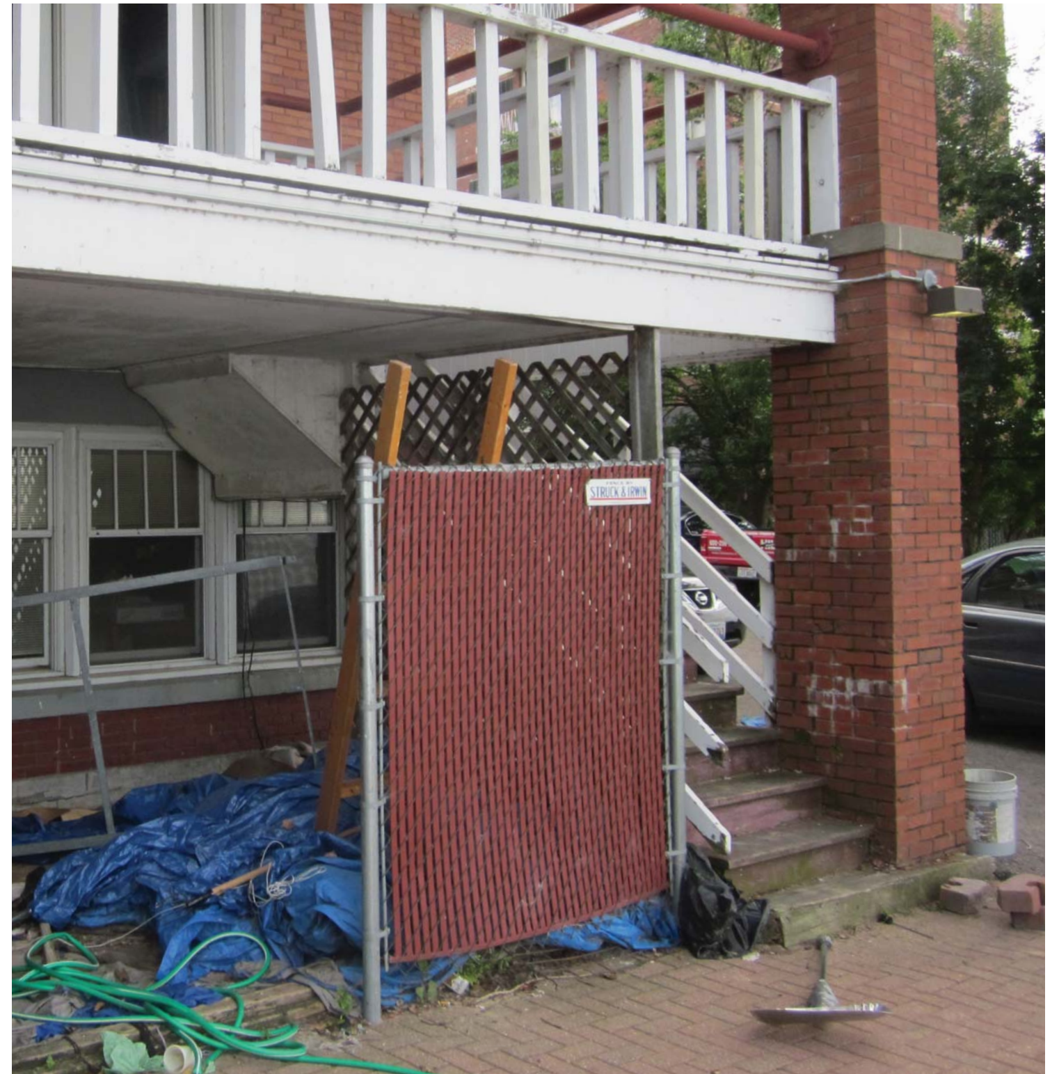
Current Conditions - Exterior - Lakefront Facade
