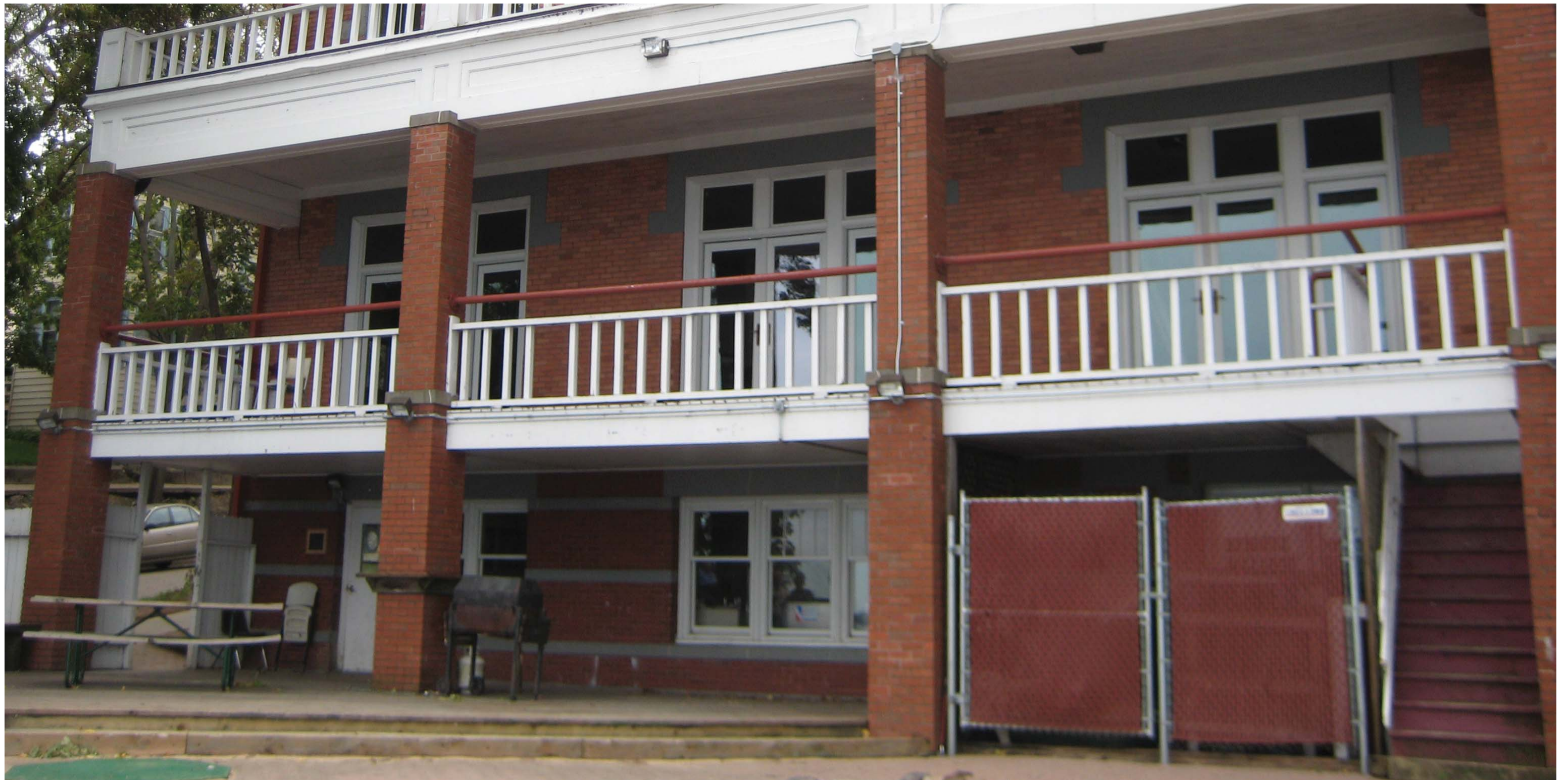
Current Conditions - Exterior - Lakefront Facade
