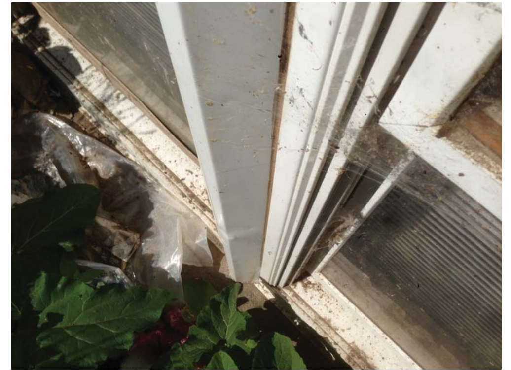
Current Conditions - Windows
