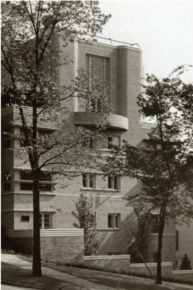
IMAGE 10: The Quisling Towers Apartments at 1 East Gilman Street, 1940. Courtesy of the Wisconsin Historical Society.
