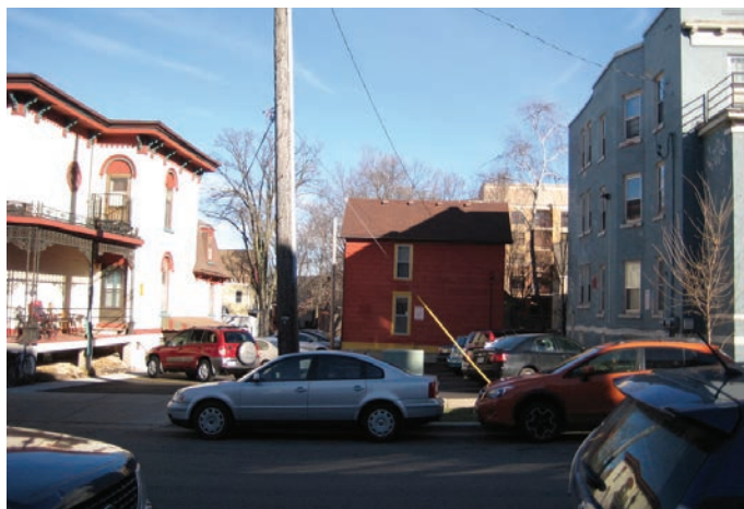
IMAGE 24: The house at 209 North Pinckney Street was razed and is now a parking lot.
