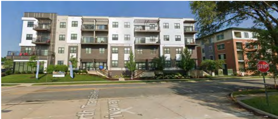
Building Across: 1201 Huxley St
