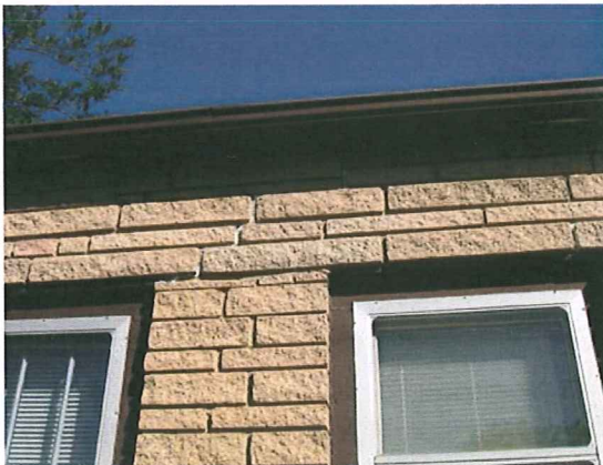
Caulking within mortar joints to attempt to repair cracking
