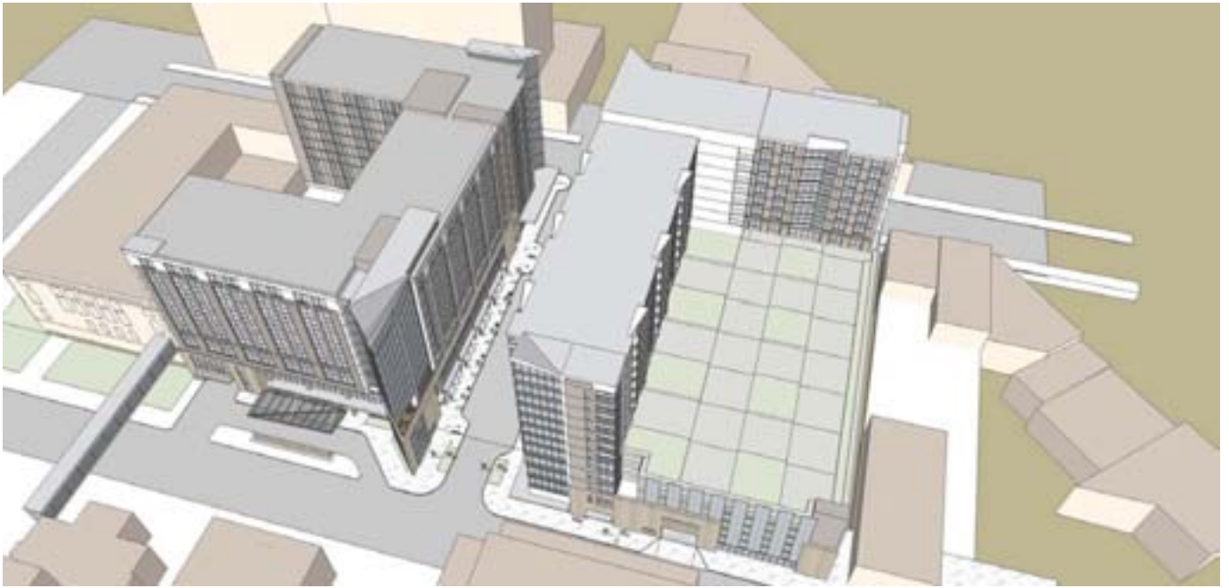
Aerial to North
