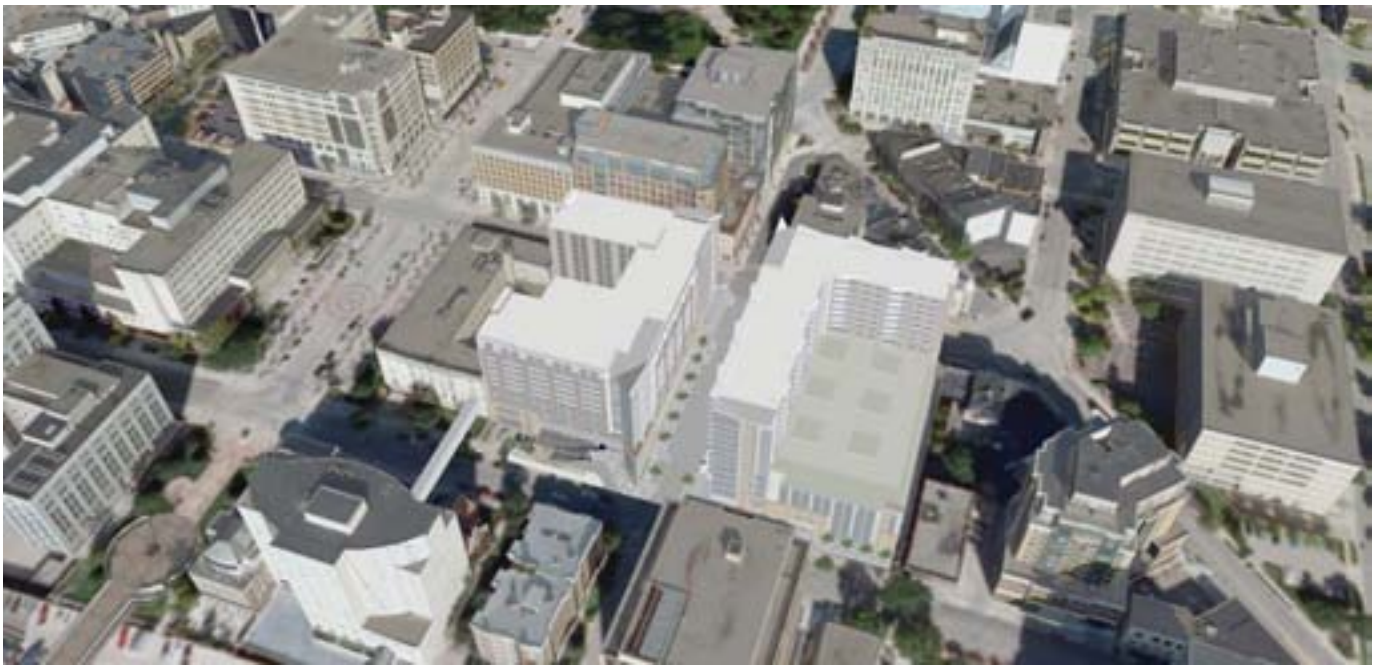
View from the West
