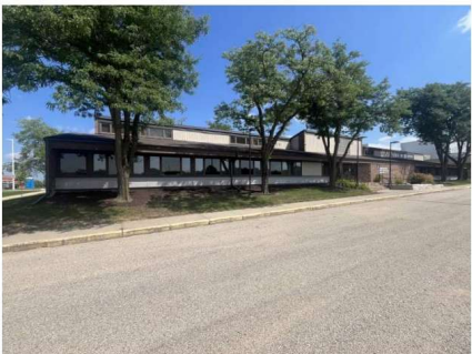
E. DANE COUNTY DEPARTMENT OF PUBLIC WORKS (ADMIN BUILDING)
