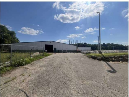
H. DANE COUNTY PUBLIC WORKS STORAGE (TO BE DEMOLISHED)
