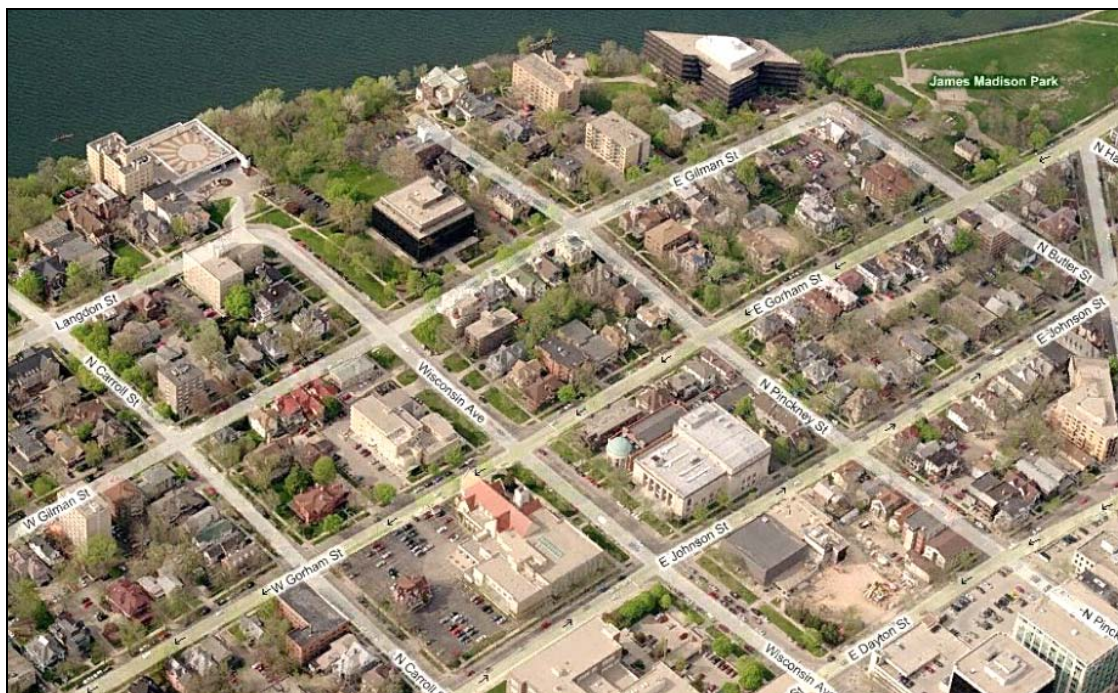
Figure 1.10 Aerial View of Existing Edgewater Hotel and Surrounding Context
