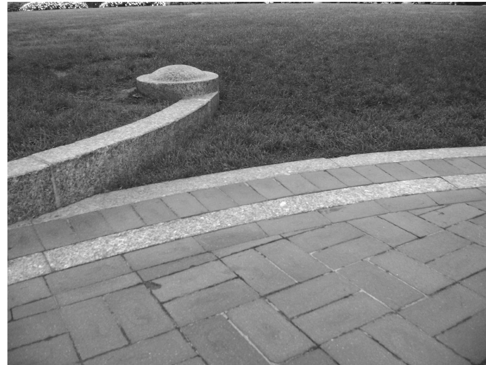
4 Lawn with Granite Curb and Brick Paving with Granite Trim Details SCALE: N.T.S.
