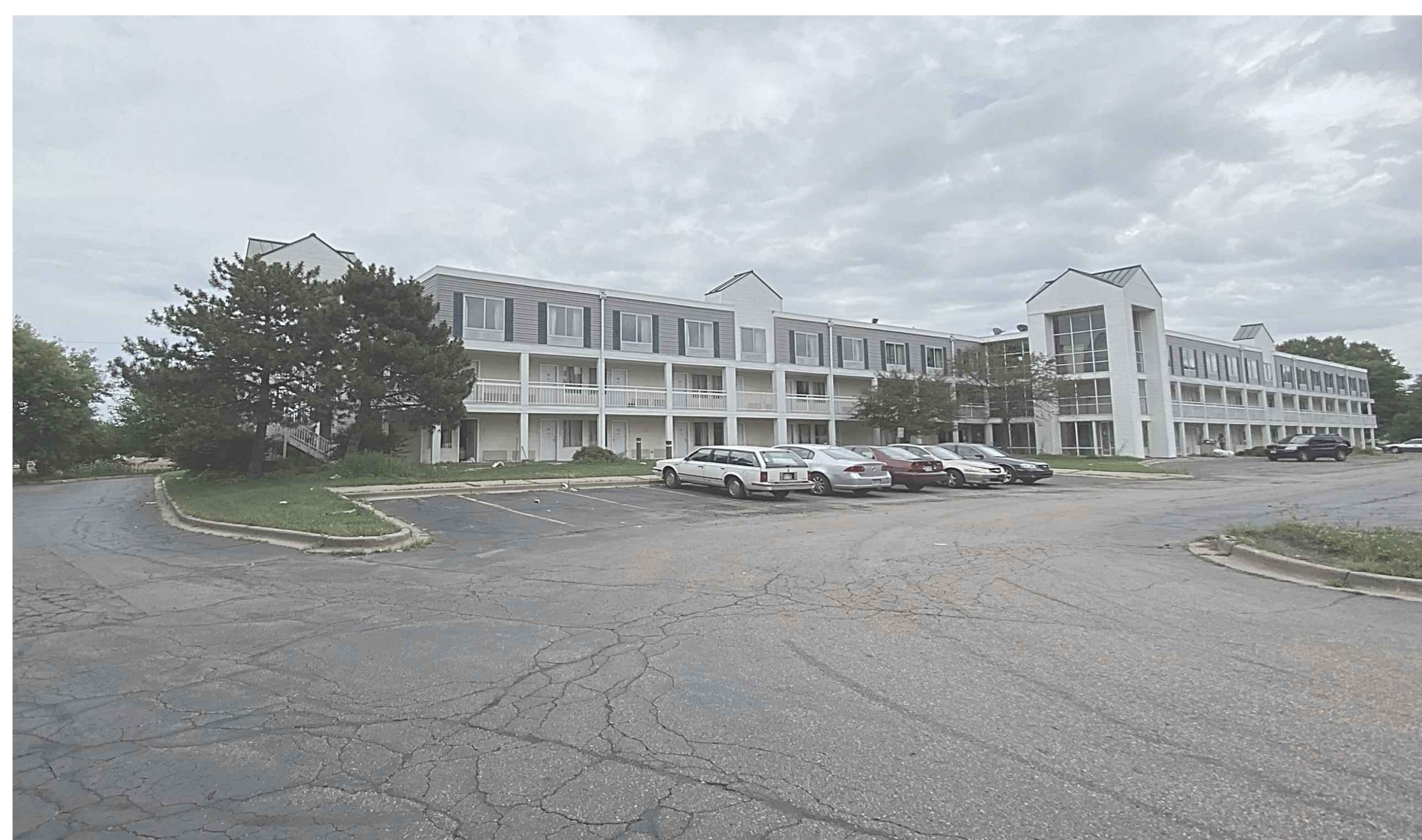
EXISTING BUILDING - LOOKING SOUTH EAST
