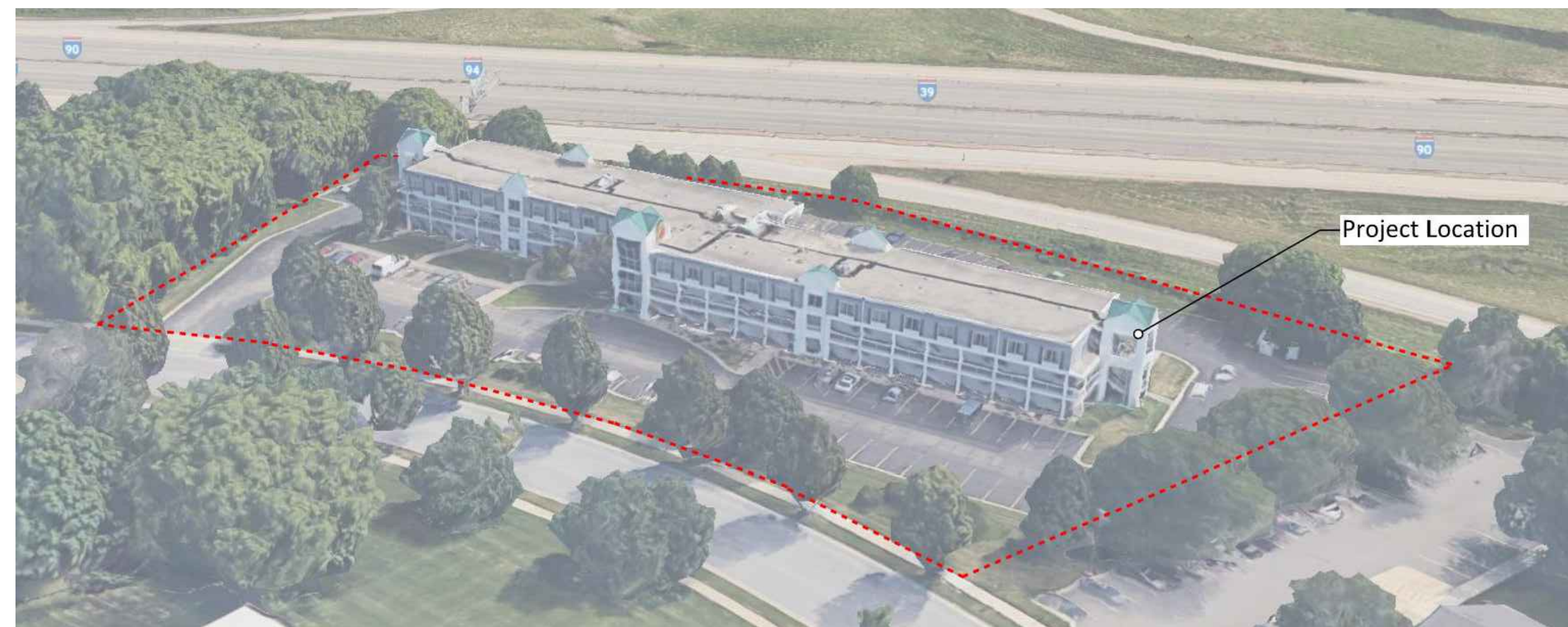
EXISTING AERIAL OF SITE - LOOKING EAST
