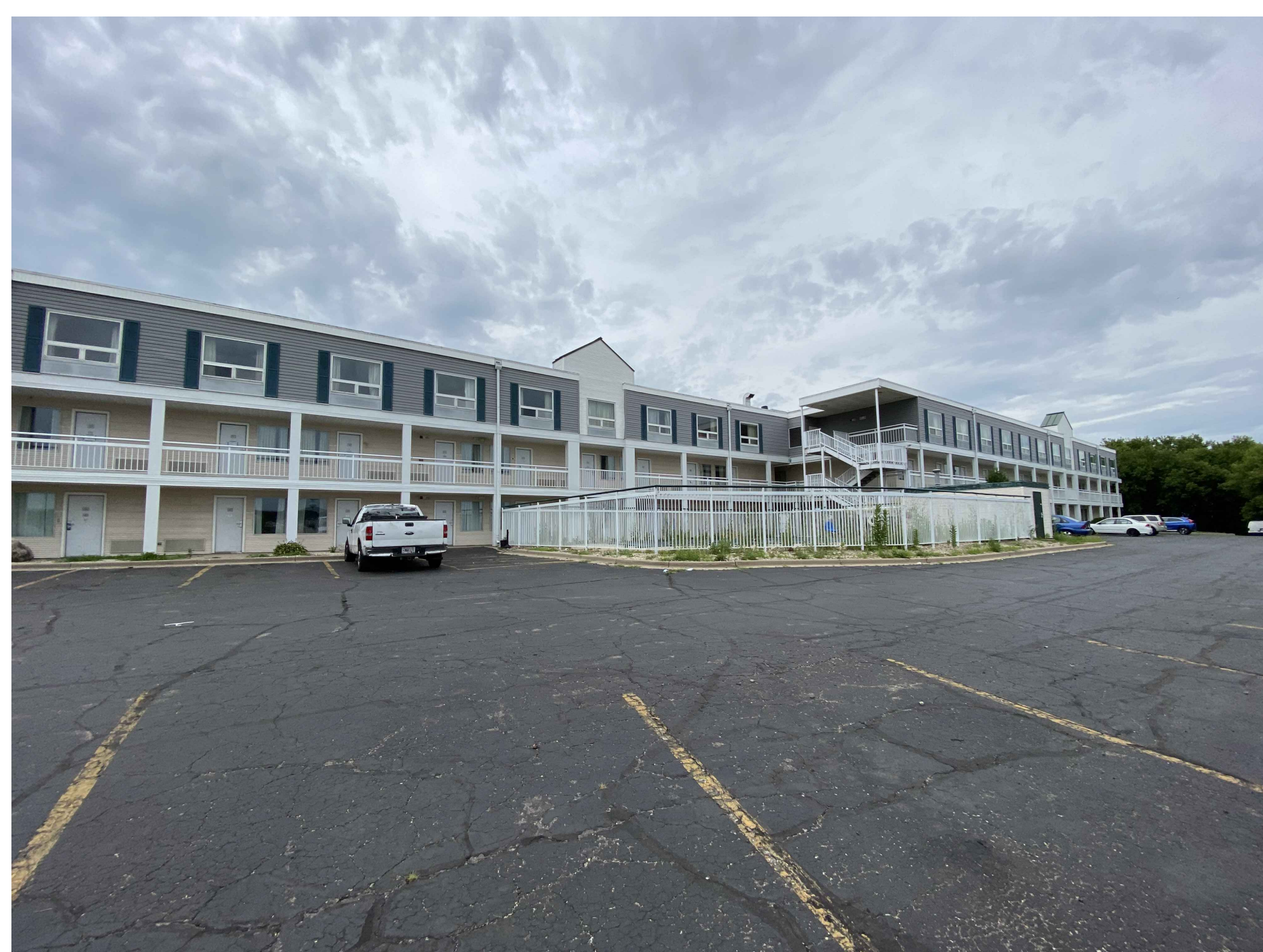
EXISTING BUILDING - LOOKING NORTH WEST
