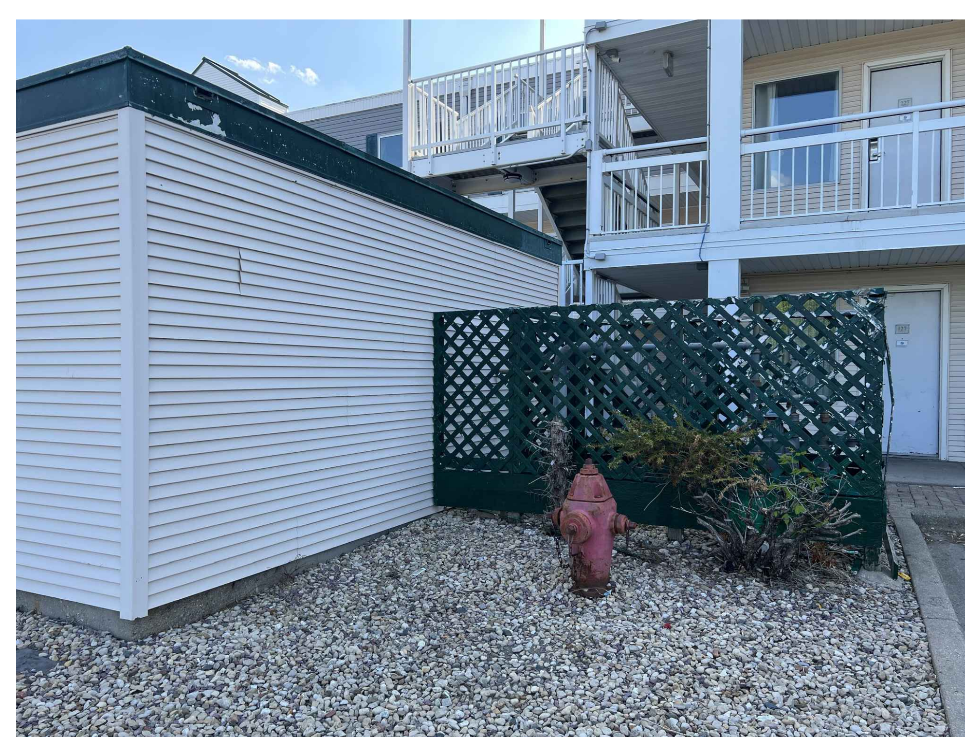
EXISTING UTILITY SCREENING - LOOKING WEST
