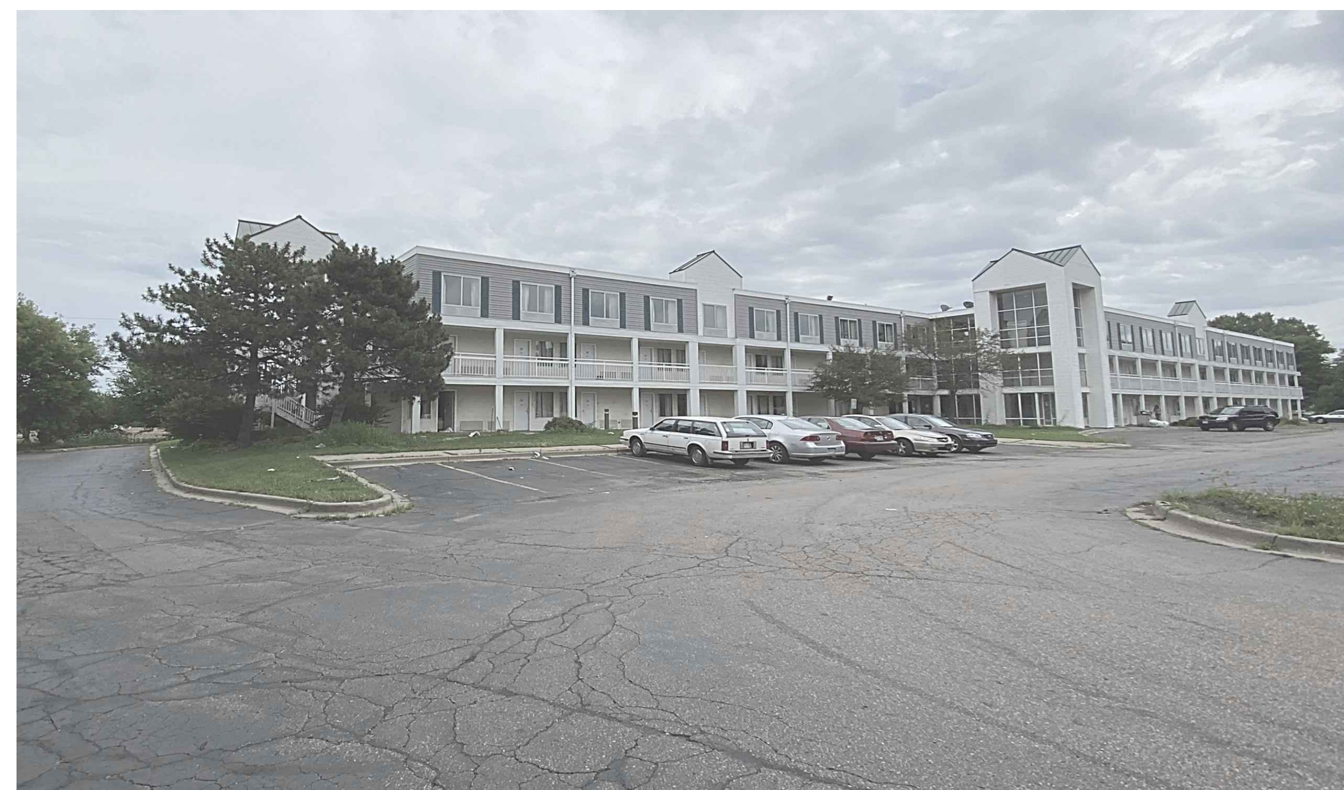
EXISTING BUILDING FACADE
