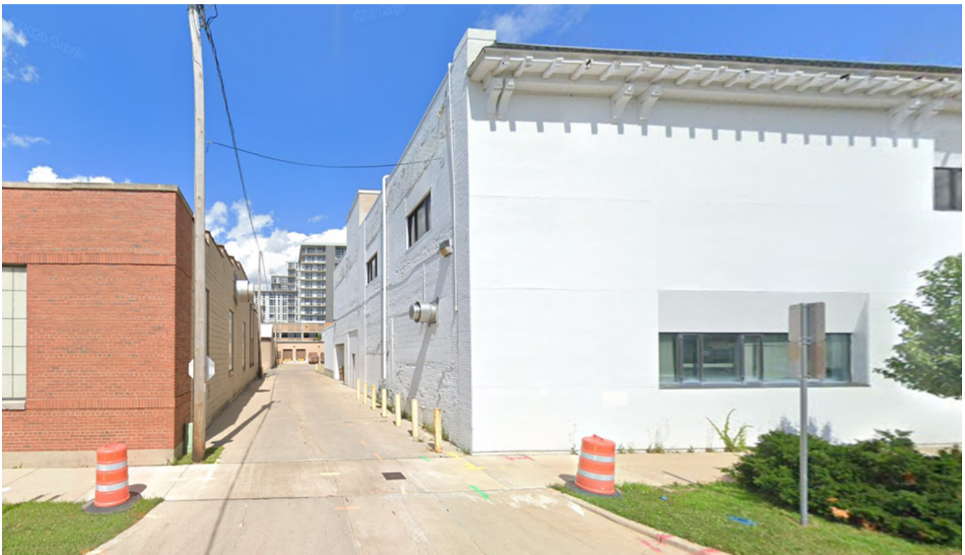
702 East Washington Avenue (White Building Only) Looking southeast down shared driveway
