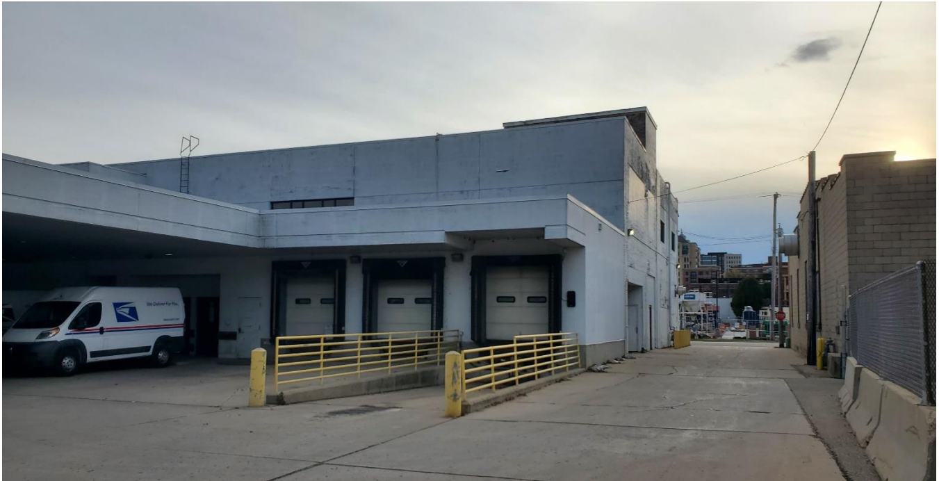
702 East Washington Avenue (White Building Only) Looking northwest down shared driveway. Vehicle canopy at left of photo.
