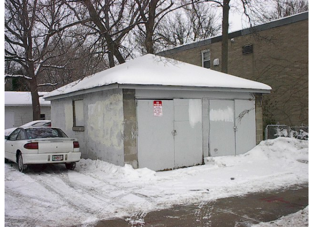
Masonry garage on 101 N. Franklin Lot to be demolished.
