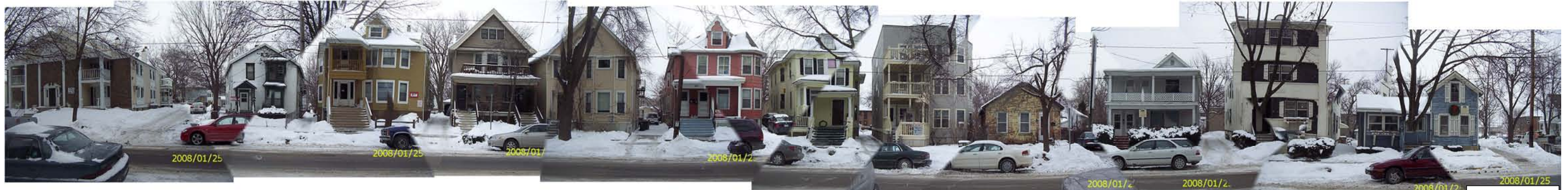
3 – North Franklin Street (East Side)
