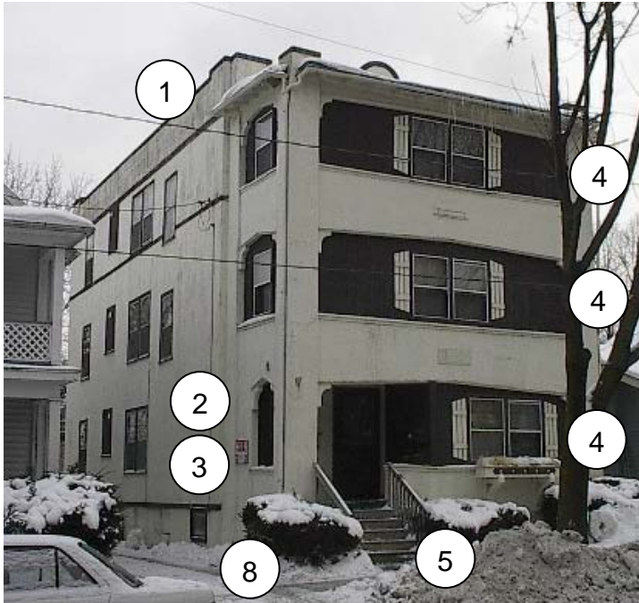
Northwest and Southwest Elevations (Front)
