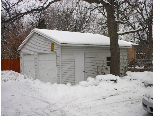
Wood-framed garage on 107/109 N. Franklin Lot to be dismantled and stored off-site for future use.
