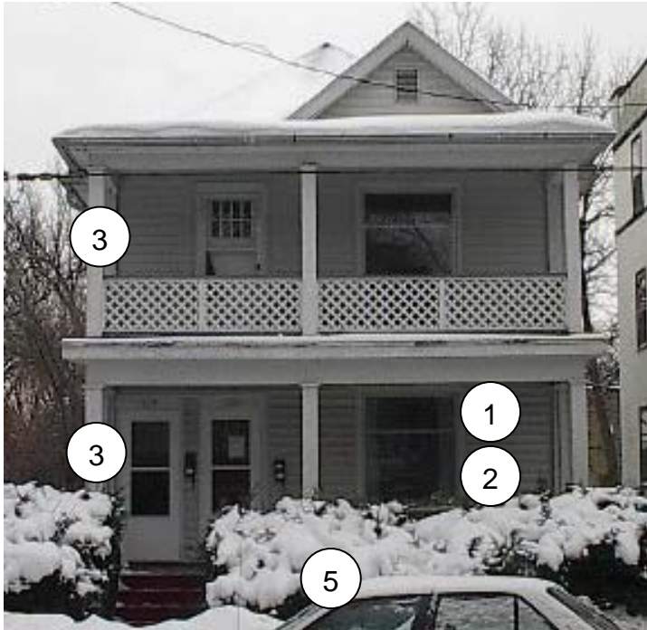
Southwest Elevation (Front)
