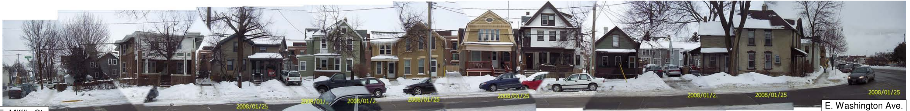
4 – North Franklin Street (East Side)
