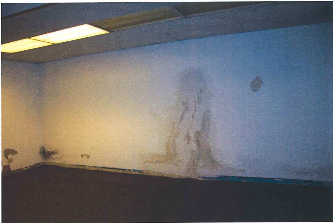
Wall in the basement
