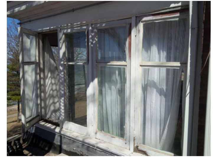
EXISTING WEST WINDOWS BEING RESTORED
