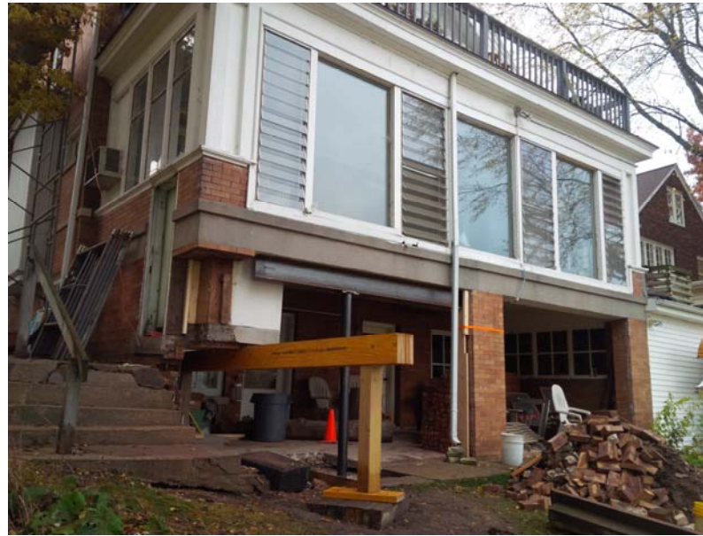
VIEW FROM PARK DURING COLUMN RECONSTRUCTION FALL 2014
