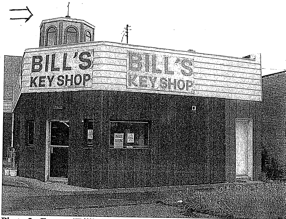
Photo 2: Former "Bill's Key Shop" facing north, note Church in background.
