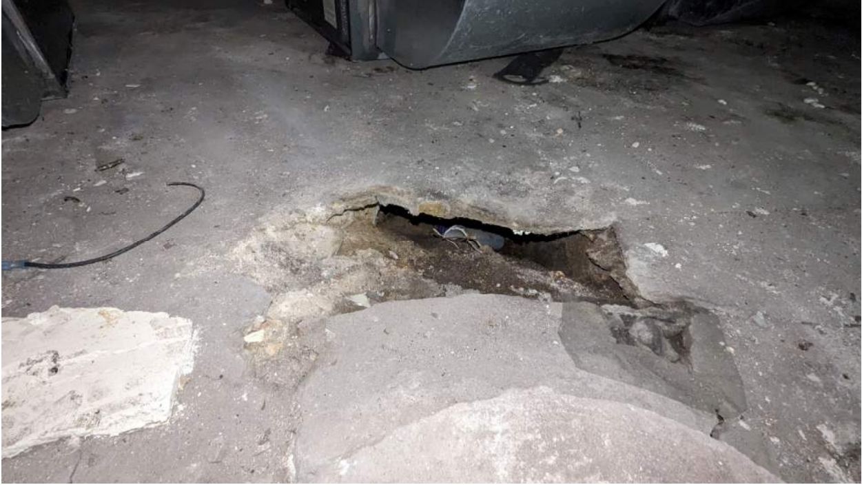
Photo 2: Large hole in basement's concrete slab-on-grade.
