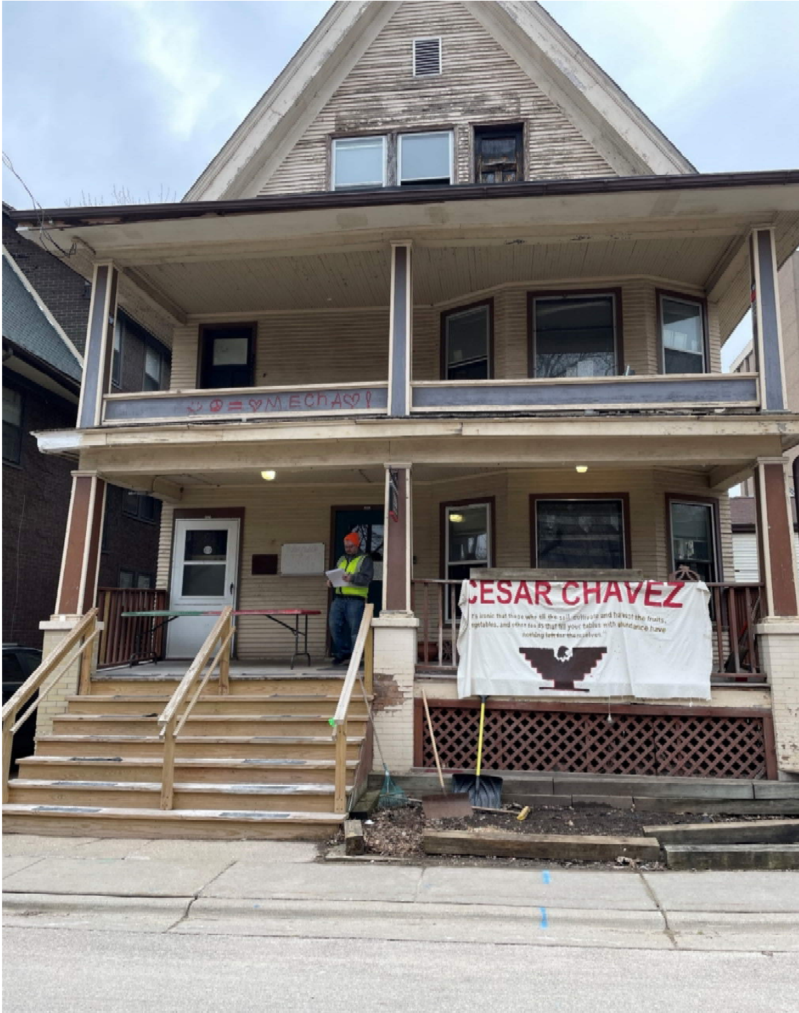
Photo 7: Settled deck and balcony with slanted joists
