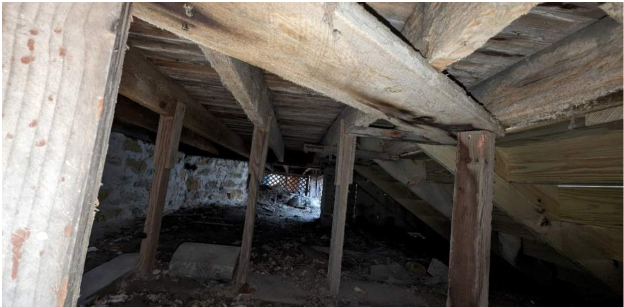
Photo 6: Temporary shoring in poor and inadequate condition underneath front deck.
