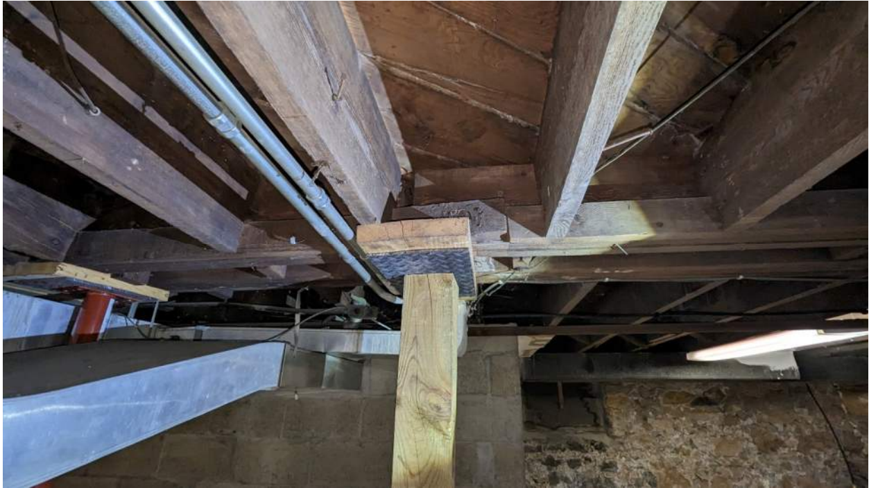
Photo 3: Unsecured temporary shoring in basement.
