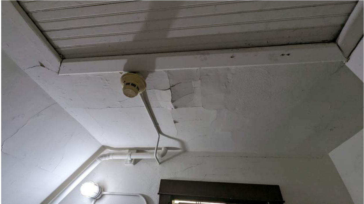
Photo 5: Minor cracking of stair ceiling.
