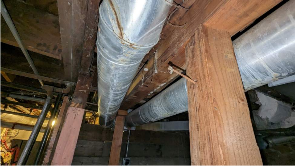
Photo 4: Unsecured temporary wood shoring in basement.
