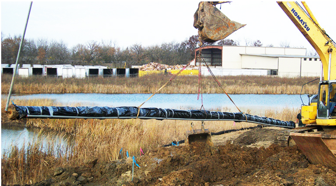
A SECTION OF THE CANNONBALL WATER PIPELINE IS INSTALLED IN SOUTH MADISON, FALL 2019
