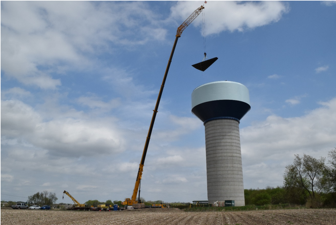
A CRANE LIFTS A SECTION OF THE STEEL ROOF INTO PLACE AT THE TOP OF BLACKHAWK WATER TOWER.
