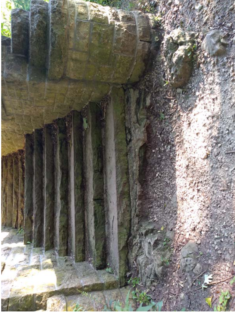
4. Existing north stairs
