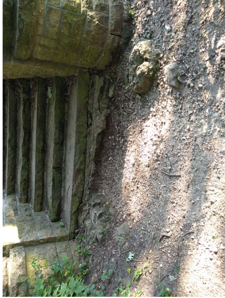
2. Existing north stairs
