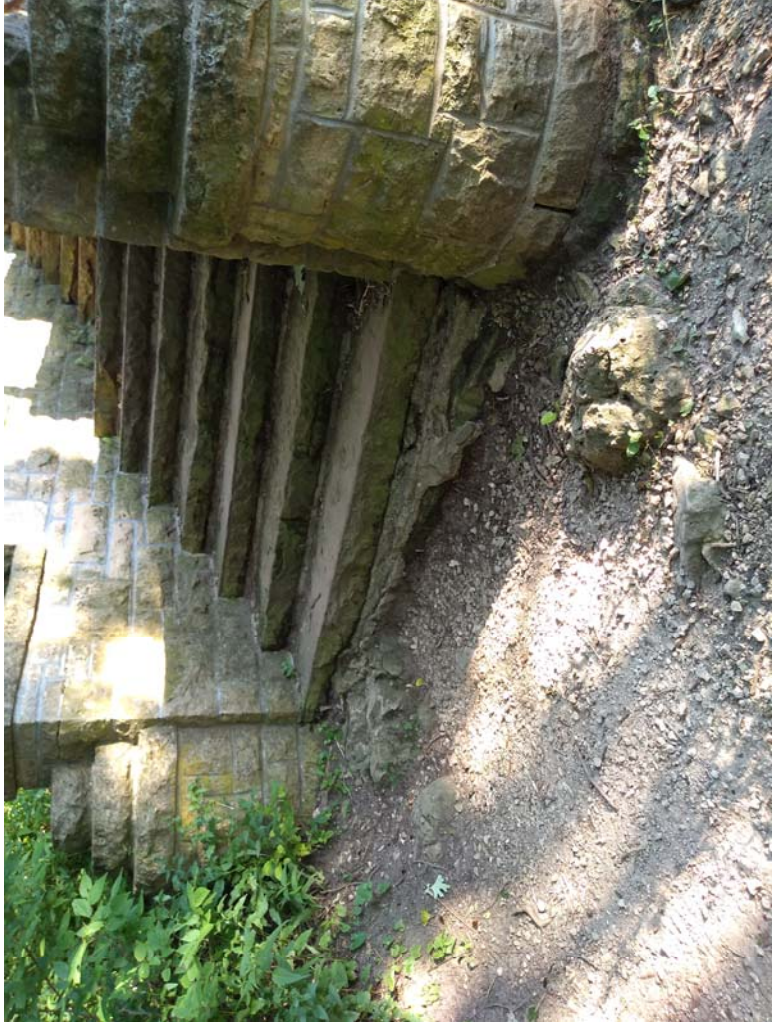
3. Existing north stairs
