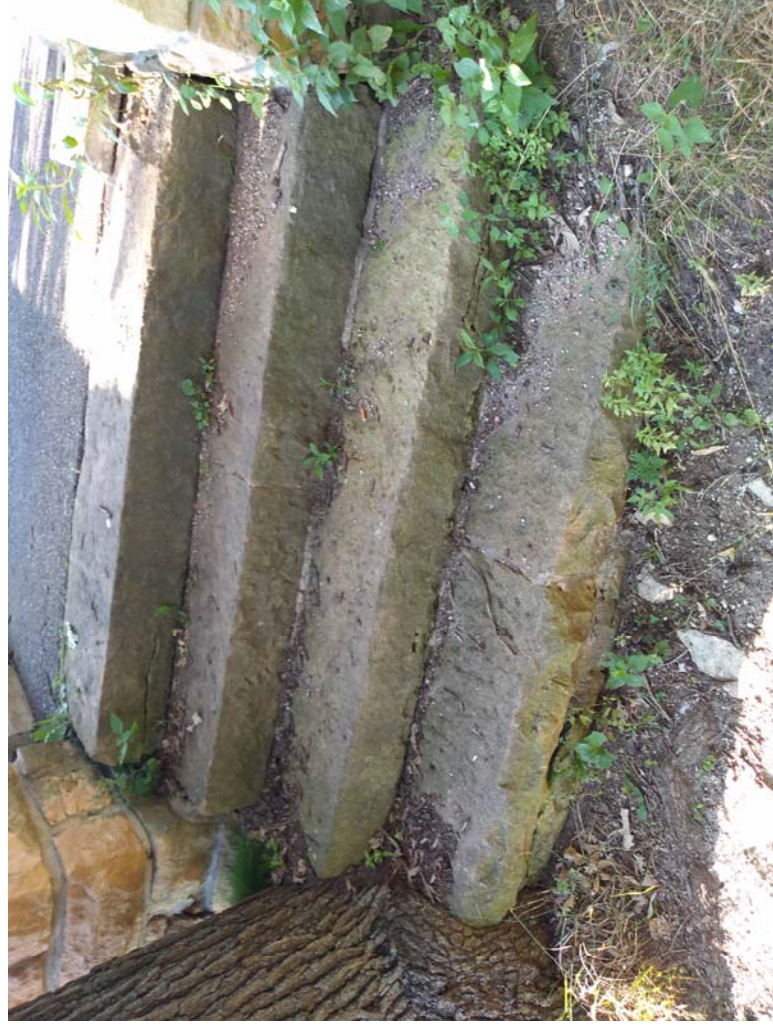
1. Existing south stairs
