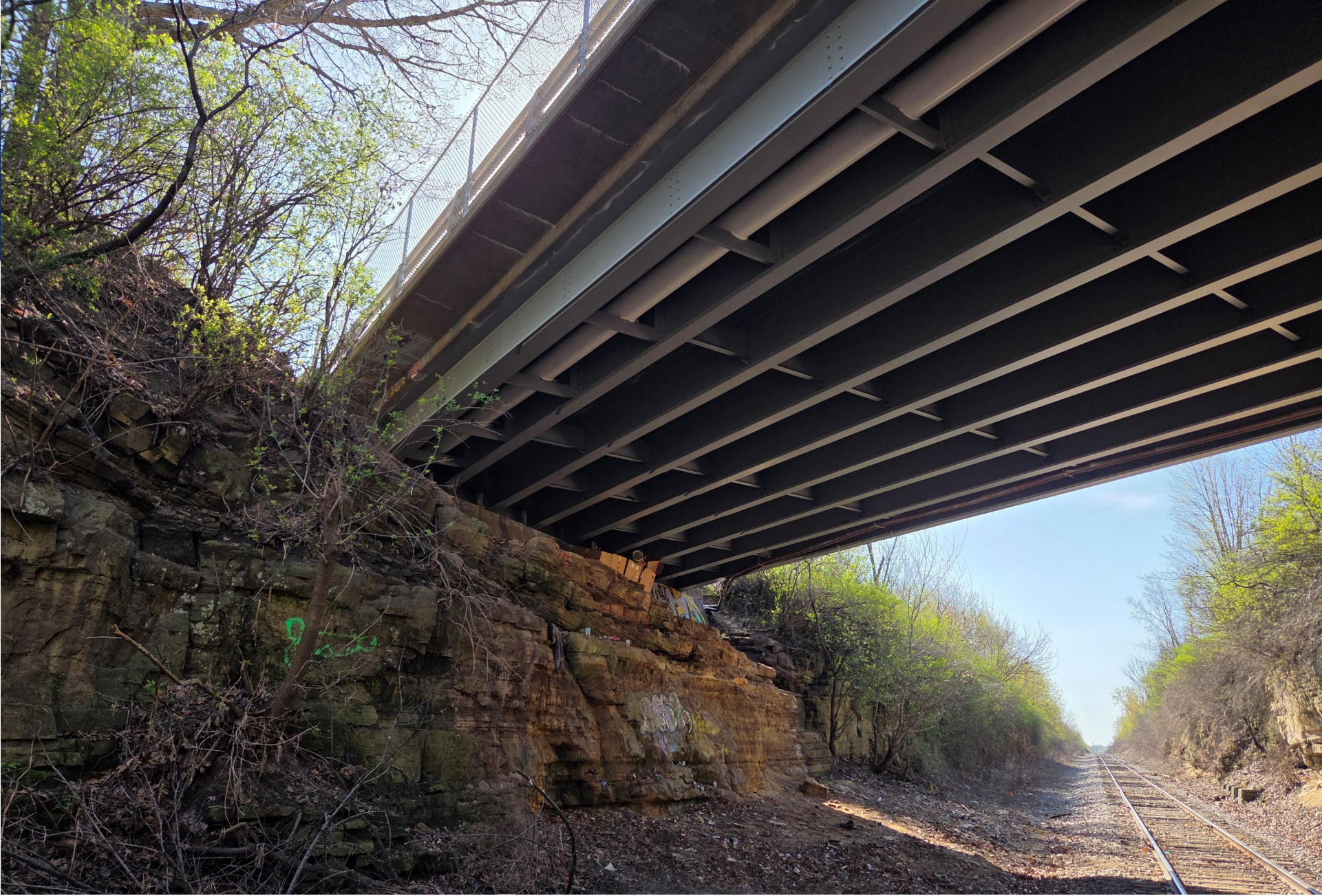
Photo: Finished Installation – Railroad Tracks Shown
