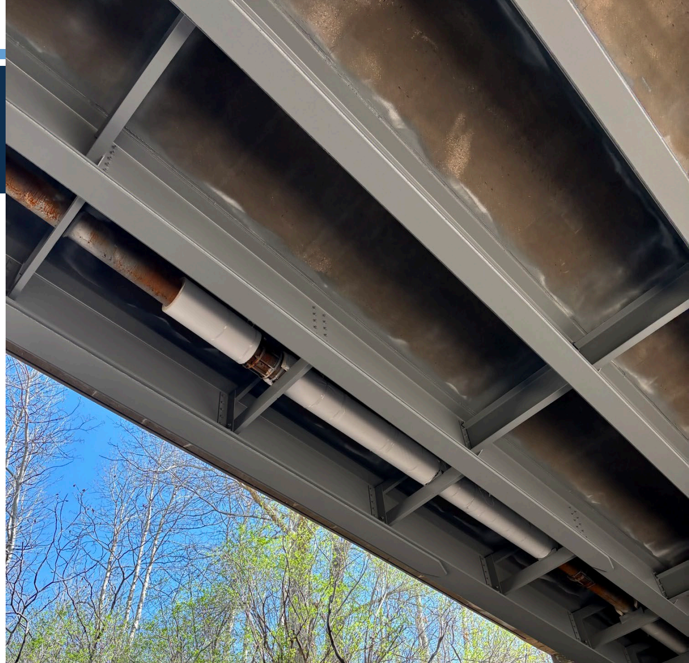
Photos: Insulation / Jacket Prep (Left) and Partial Application (Right) 56
