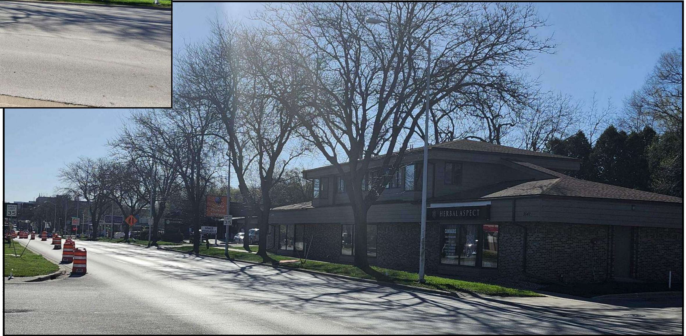
EXISTING VIEW - EAST FACING
