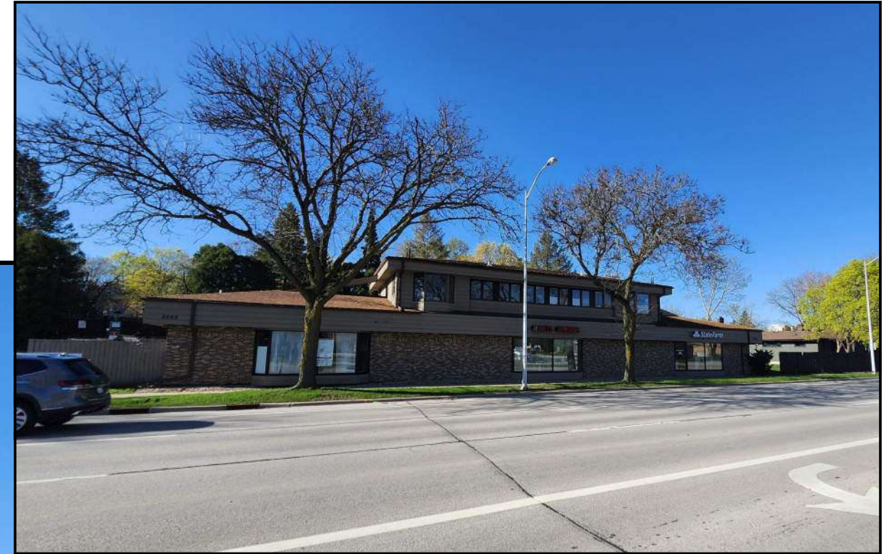
EXISTING WEST BUILDING 3553 UNIVERSITY AVENUE
