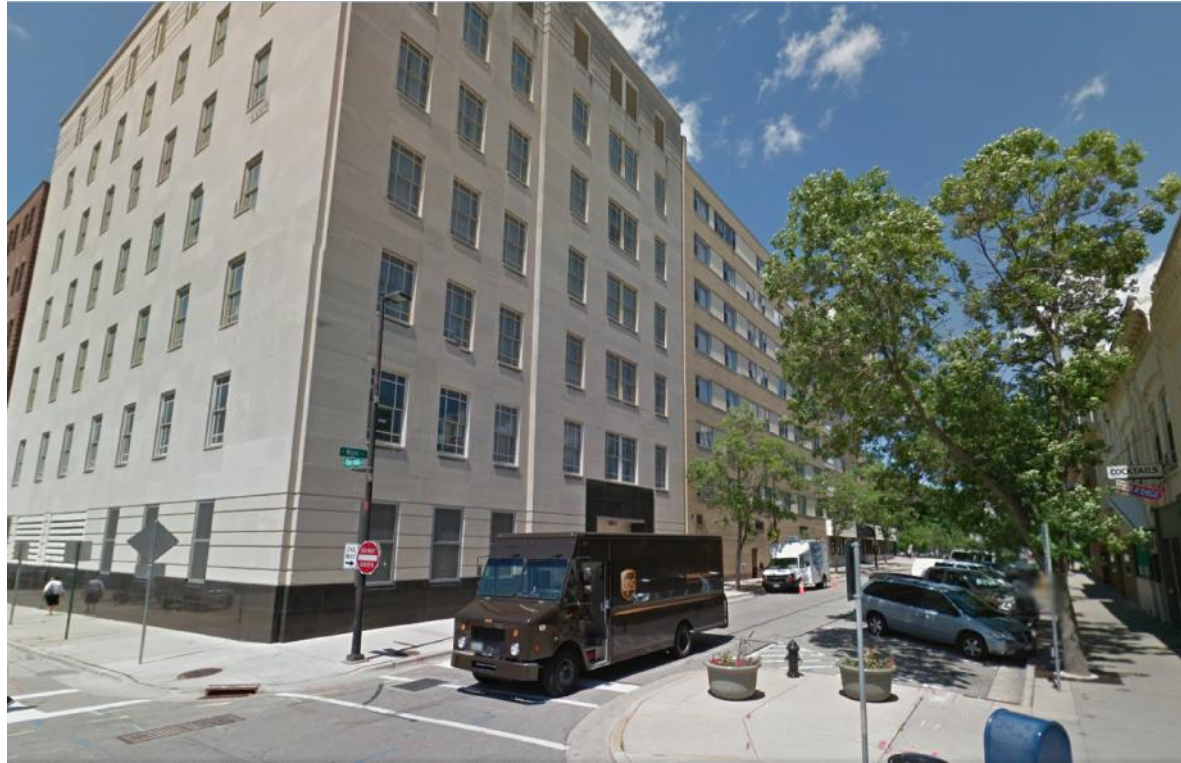
Main Street at adjacent building
