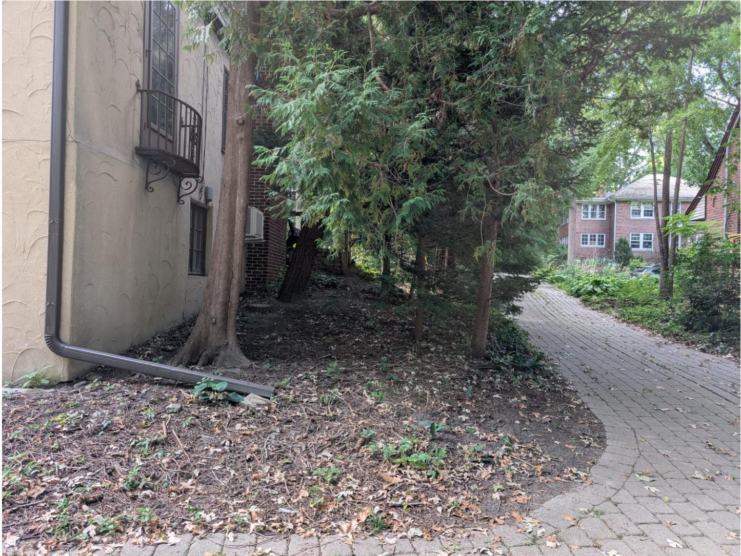
West Side Elevation, driveway, looking toward Bascom
