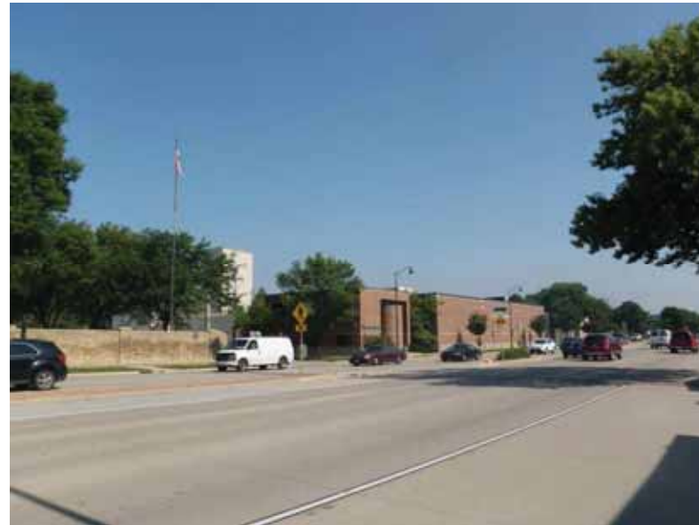
VIEW FROM EAST WASHINGTON LOOKING NORTHEAST
