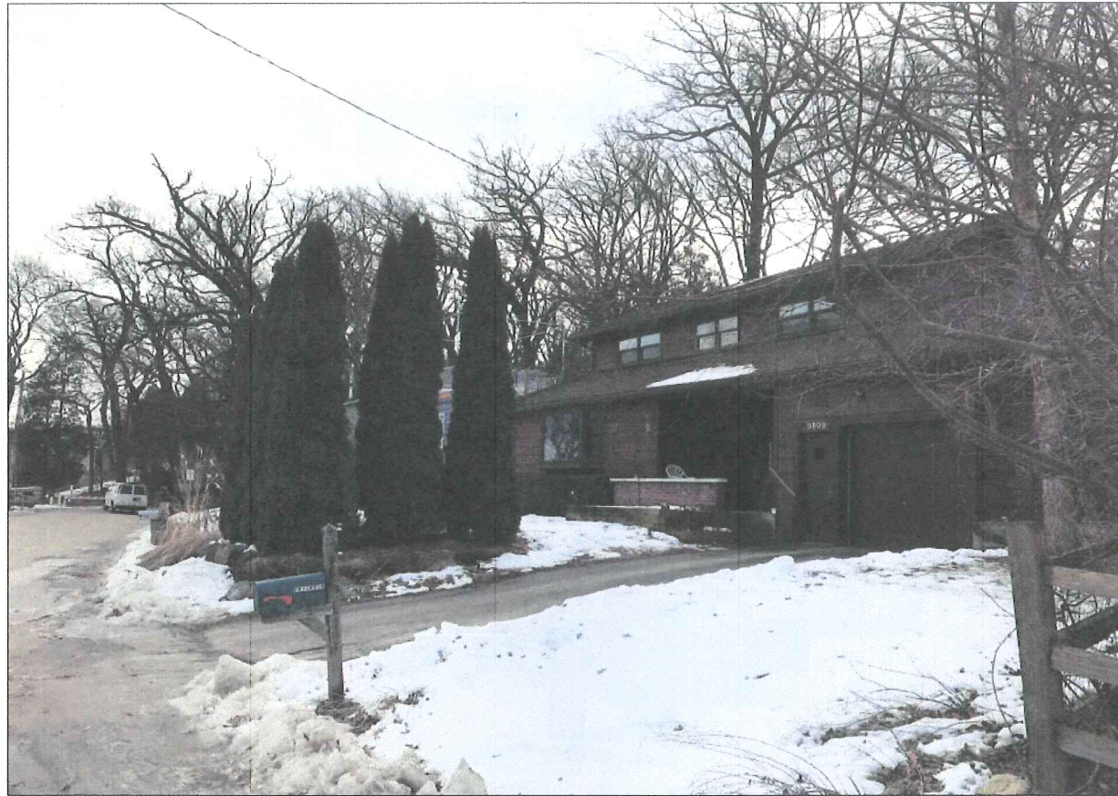
ADJACENT BUILDING SOUTH
