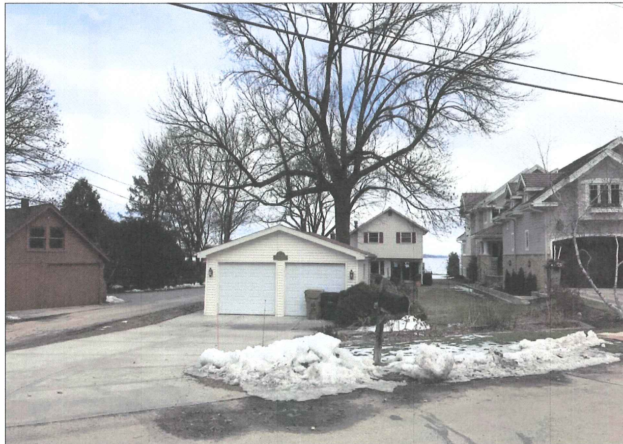
ADJACENT BUILDINGS WEST
