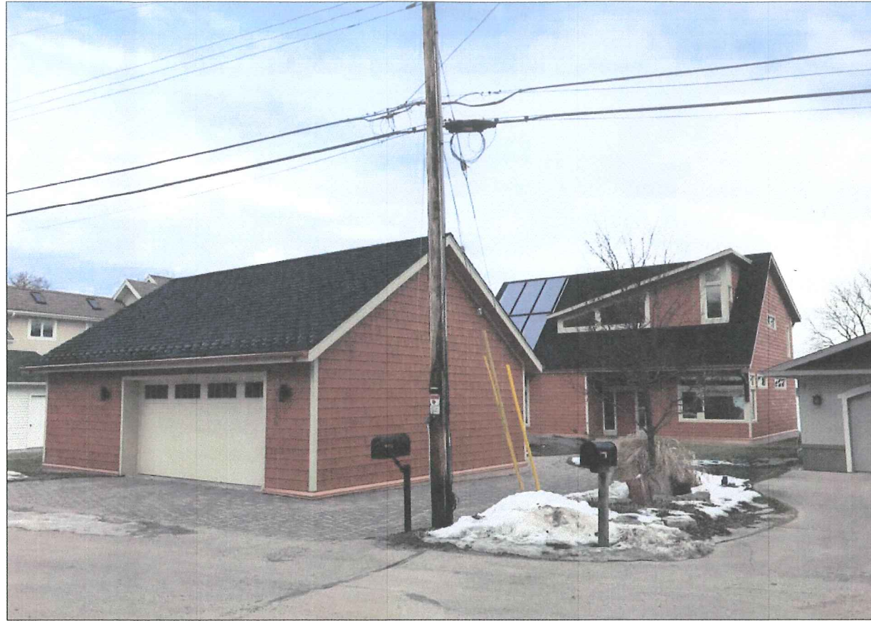
ADJACENT BUILDING EAST
