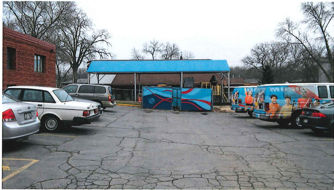
West Elevation, view from parking lot
