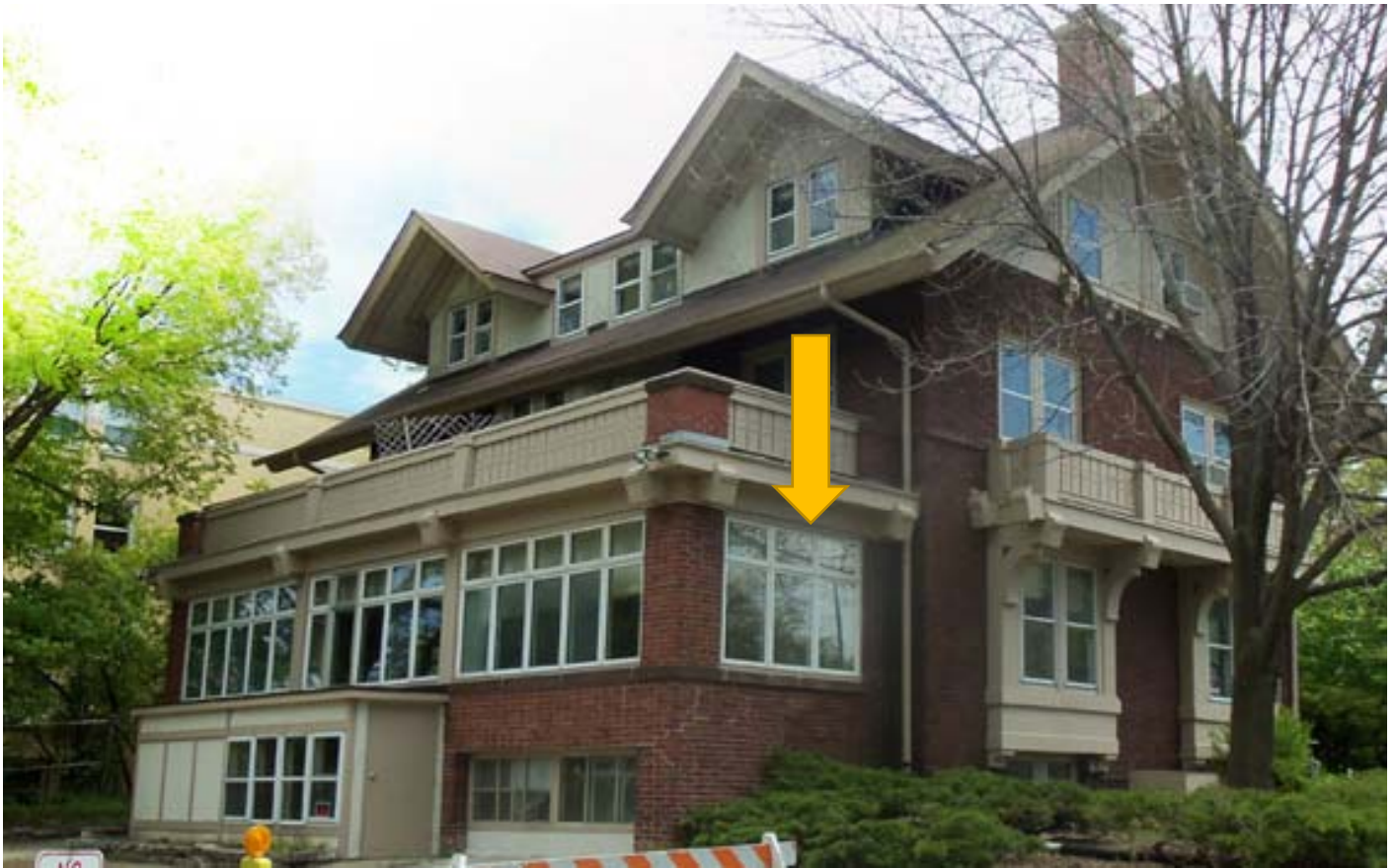
West facing side of house, replace west facing bay, current mix of fixed and casement and fixed transom.
