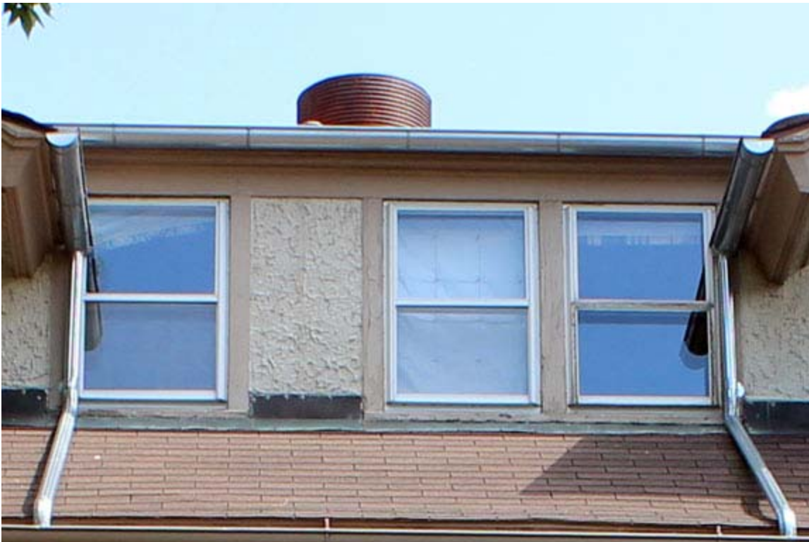
Dormer close up
