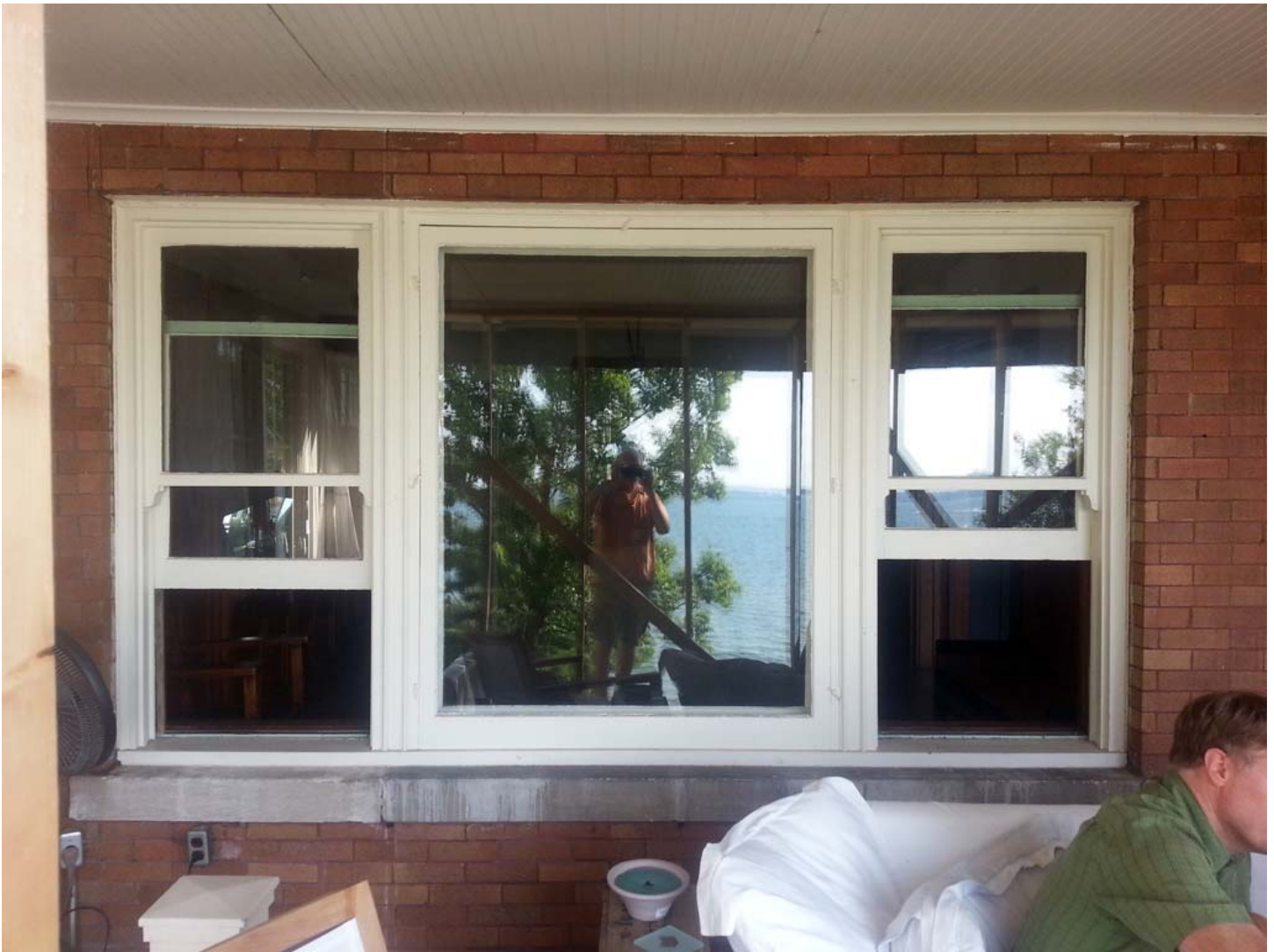
Photo of original window configuration on the back side of Claude and Stack designed home next door at 646 E. Gorham showing the picture window flanked by double hung configuration.
