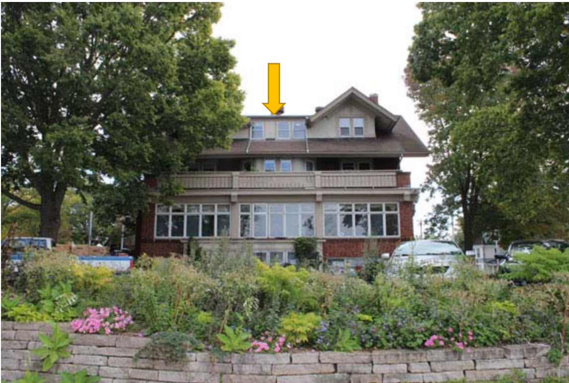
Back of house, top floor center dormer showing existing configuration of 3 double hung
