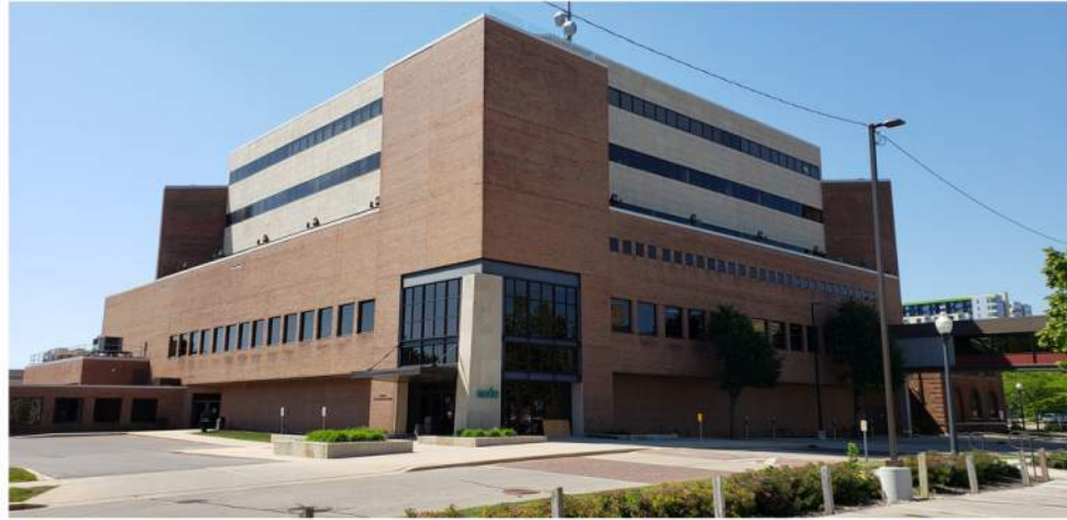
Existing MGE GOF Building
