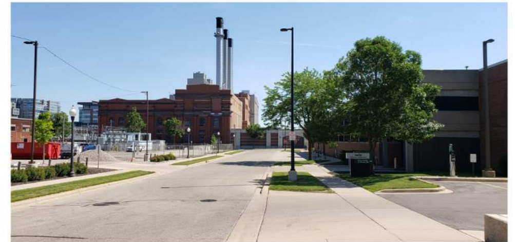
View East down Railroad Street
