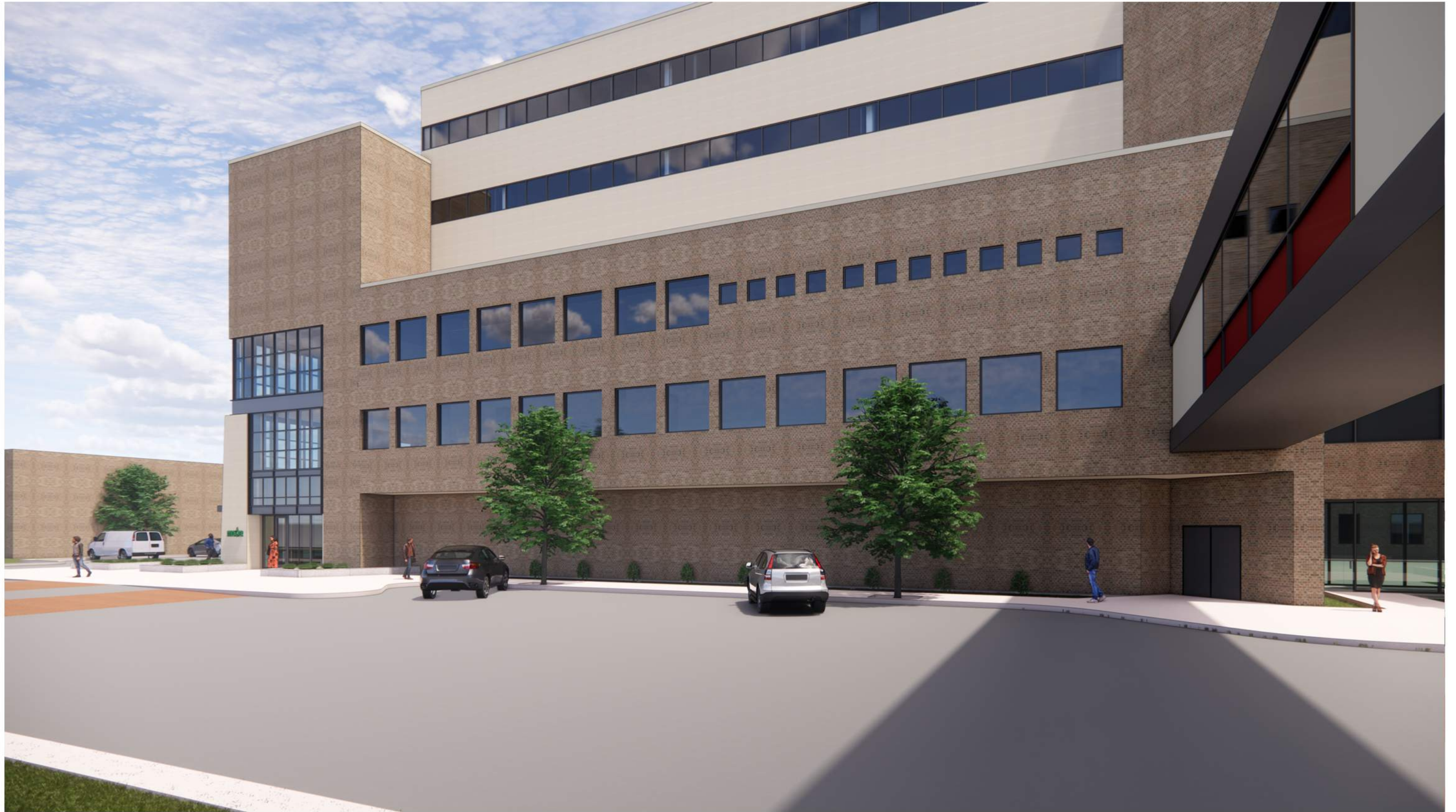
Railroad Street view
