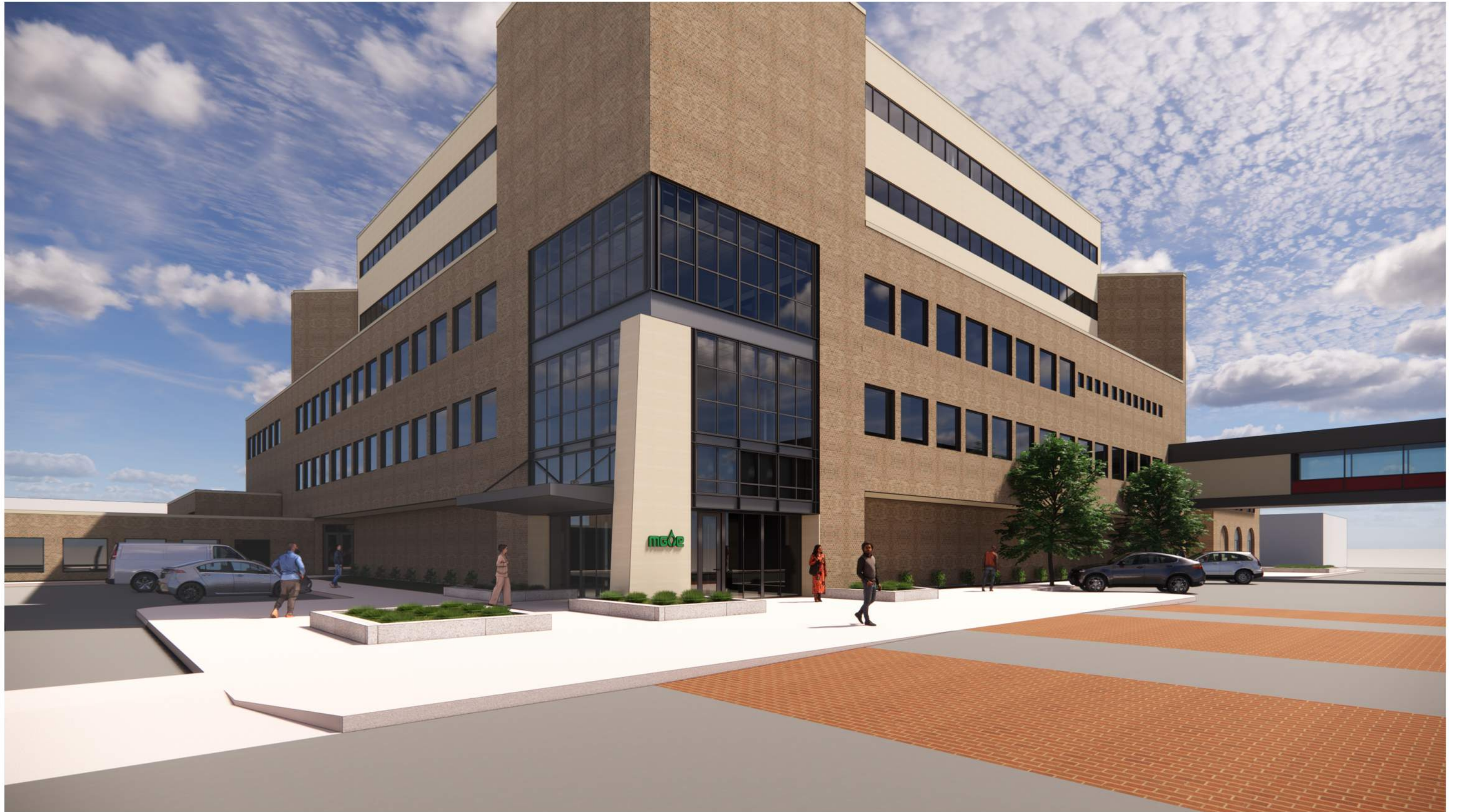
Railroad Street view - North Entry corner
