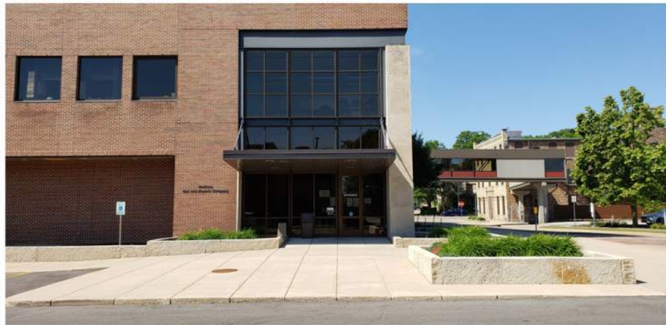
Existing MGE GOF main entry
