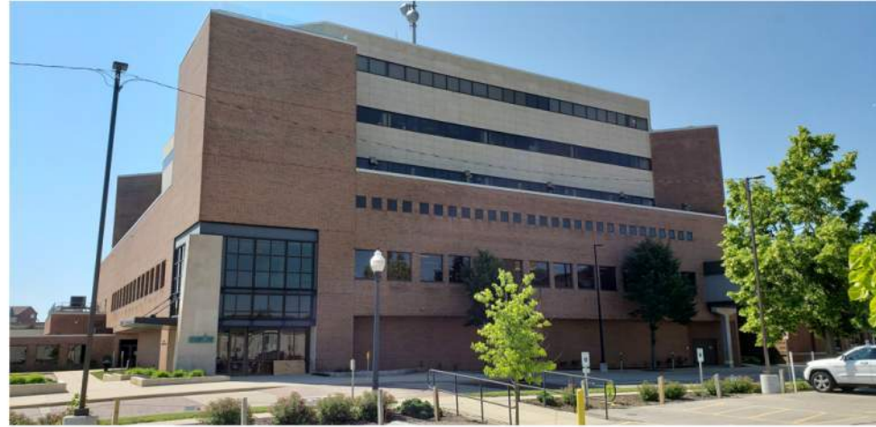
Existing GOF Building along Railroad Street
