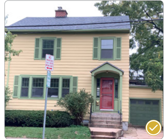
Figure 107: Compatible garage doors that share architectural qualities with the main building at 1005 Oakland Avenue (41.26.5.d.1).
