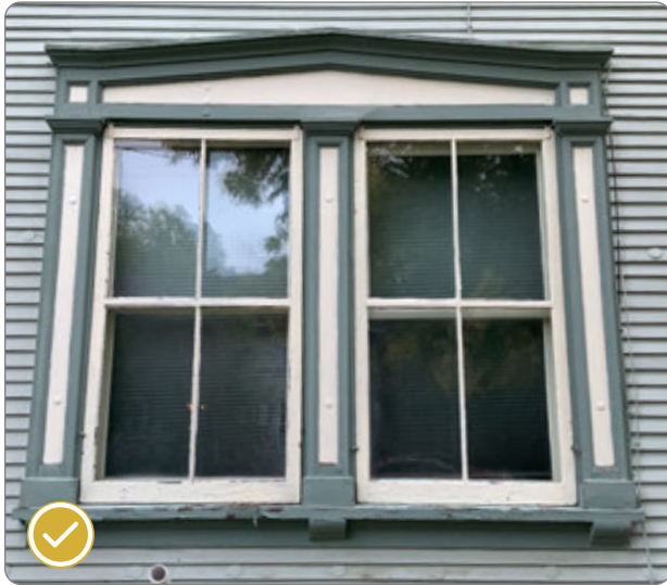
Figure 67: The left image has compatible wood framed storm windows with painted trim to match original sashes (41.25.5.c.6). The right image has incompatible reflective aluminum framed storm windows that do not blend with the historic sashes (41.25.5.c.6).
