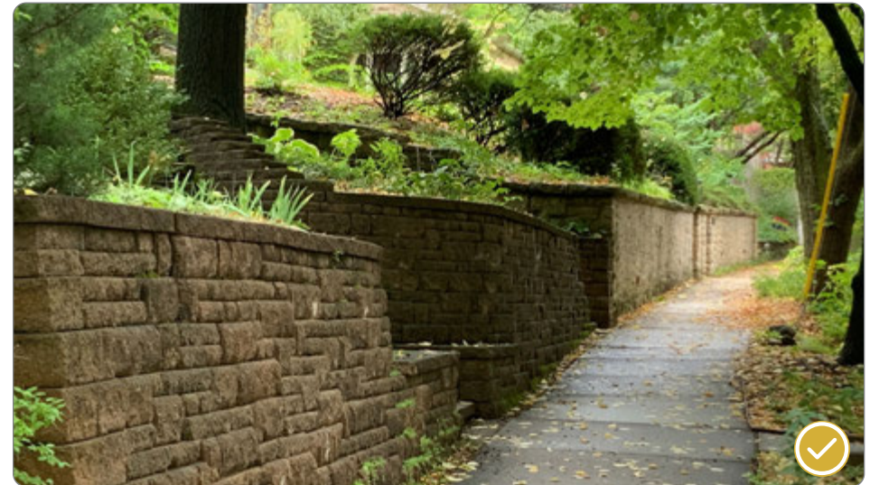
Figure 51: Retaining wall in the University Heights District.
