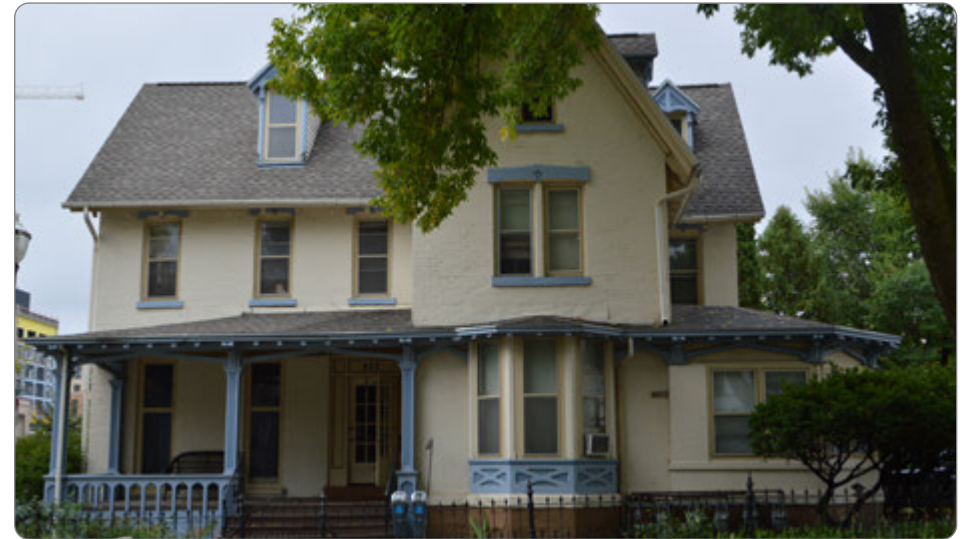
Figure 2: Example of well maintained residential building in the Mansion Hill Historic District at 422 N Henry Street.
