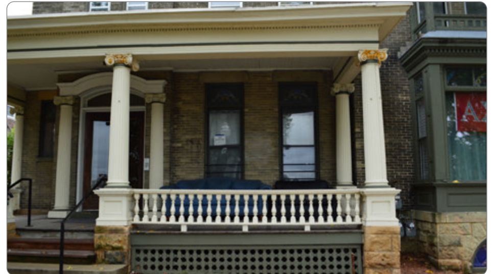
Figure 139: Porch details seen in Madison (41.27.6.a.1).
