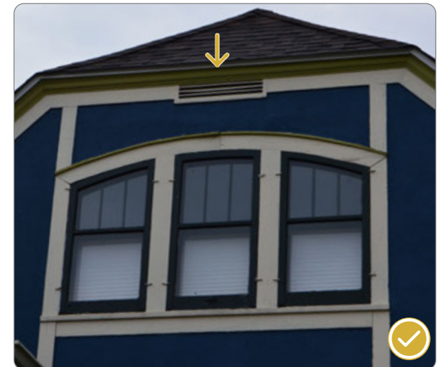
Figure 117: Vent finished and painted to match architectural trim of building (41.26.7.a.3).
