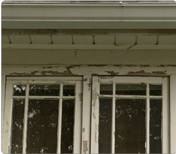
Figure 39: Wood features requiring repair (41.24.2.b.1).
