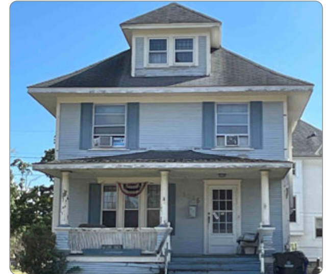
Figure 10: Moderate Integrity Building.
