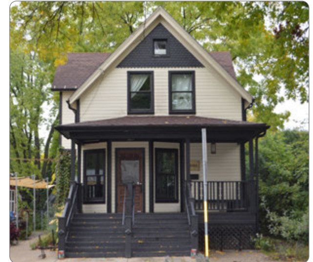
Figure 77: Example of full-width porch enclosed with lattice and with painted handrails at 1380 Williamson Street (41.25.6.b.2-4).
