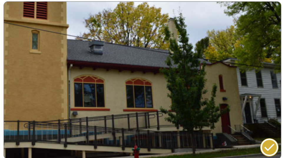
Figure 49: Compatible accessibility ramp constructed on side of historic public building at 504 S Breatly Street (41.25.1.d.2).
