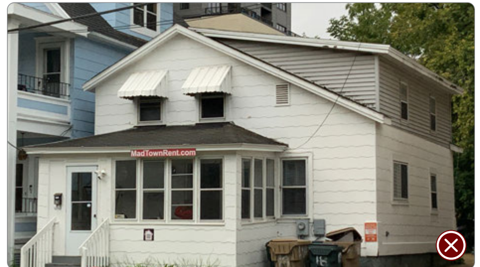
Figure 101: Incompatible dormer addition to residence (41.26.4.f.1-4).
