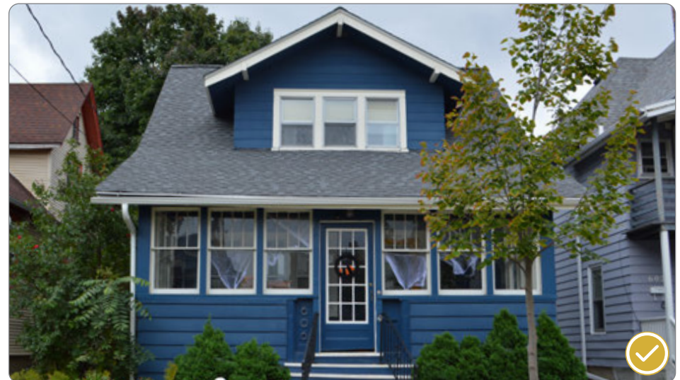
Figure 80: Enclosed porch at 606 S Baldwin Street (41.25.6.c.1).
