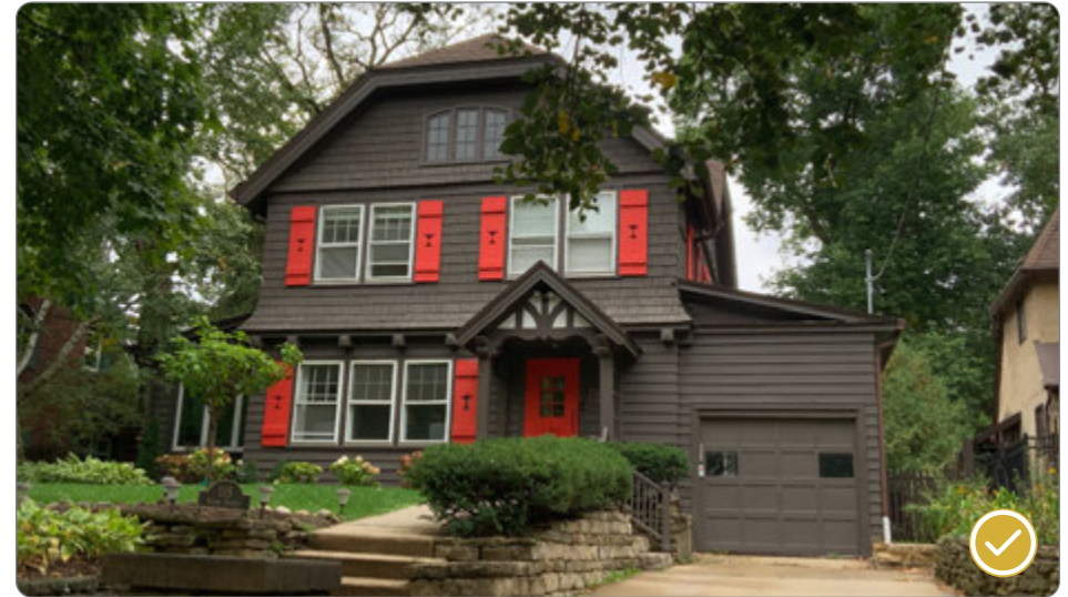
Figure 93: Side addition on a residential building at 115 North Allen Street (41.26.3.a.1).
