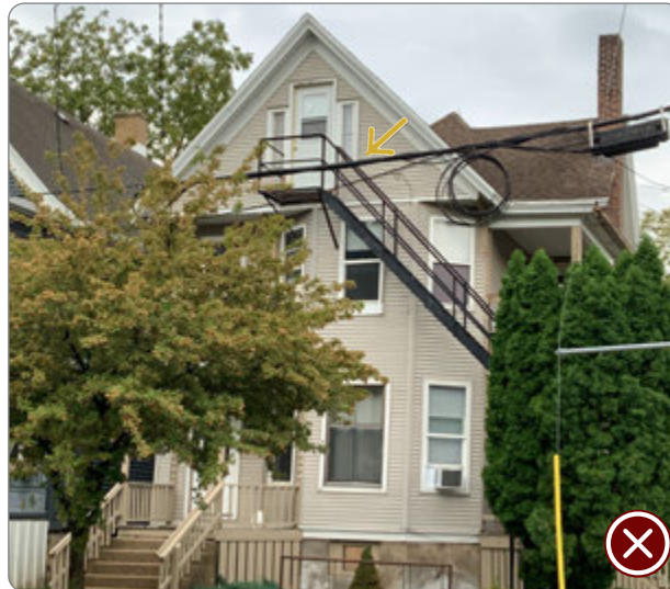
Figure 109: Example of a second exit stairway off the front of the building (41.26.6.a.4).
