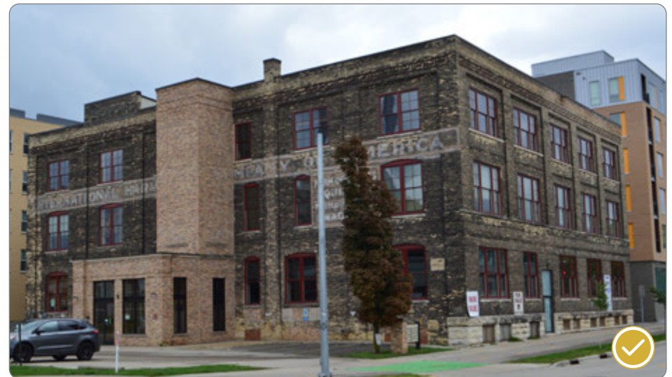
Figure 88: Side addition on a public building that is compatible but visually distinct at 301 S Blount Street (41.26.1.a.2-4).
