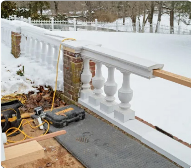
Figure 32: Oatlands Plantation Leesburg, Va., the National Trust for Historic Preservation tested acetylated wood on this weather-prone balustrade.
