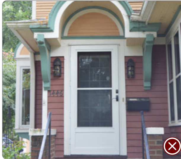
Figure 106: Incompatible storm door, new storm doors need to be full light (41.26.5.d.1).
