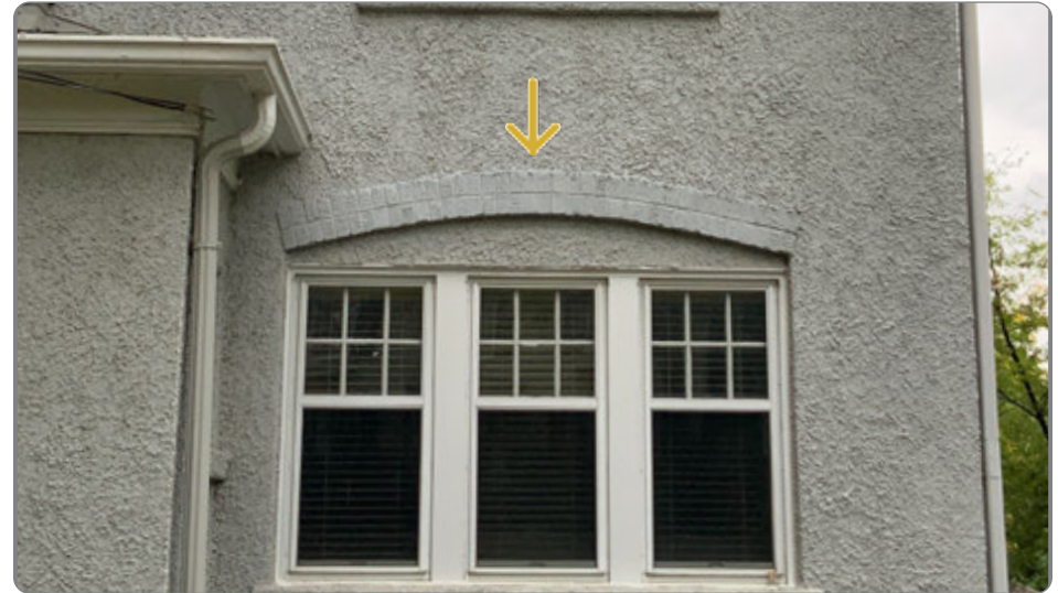
Figure 63: Infilled head above windows (41.25.5.b.1).
