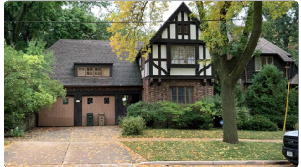
Figure 96: Compatible roof pitch and form on side addition at 1608 Adams Street (41.26.4.a.1).
