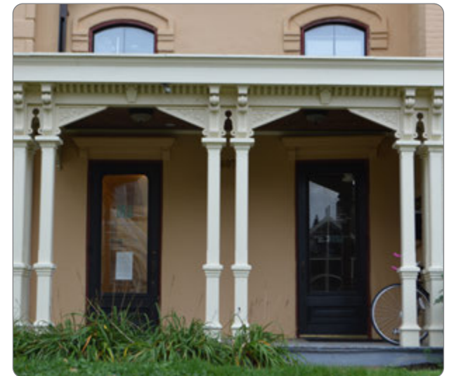
Figure 40: Wood porch details in good condition (41.24.2.b.1).
