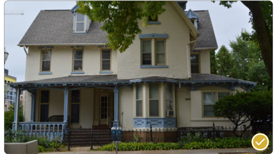
Figure 50: Compatible front yard fence at 422 N Henry Street.
