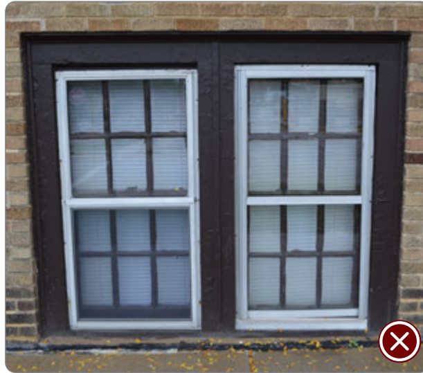
Figure 67: The left image has compatible wood framed storm windows with painted trim to match original sashes (41.25.5.c.6). The right image has incompatible reflective aluminum framed storm windows that do not blend with the historic sashes (41.25.5.c.6).
