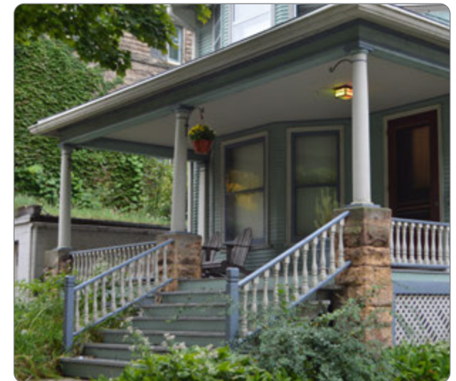
Figure 31: Well preserved porch at 28 S Franklin Street (41.23.4.a.1).
