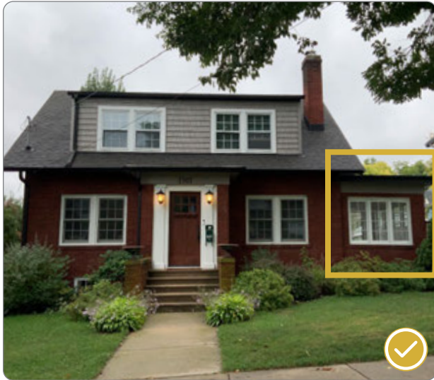
Figure 102: Addition windows that are compatible with the historic building at 1707 Madison Street (41.26.5.1.a-b).
