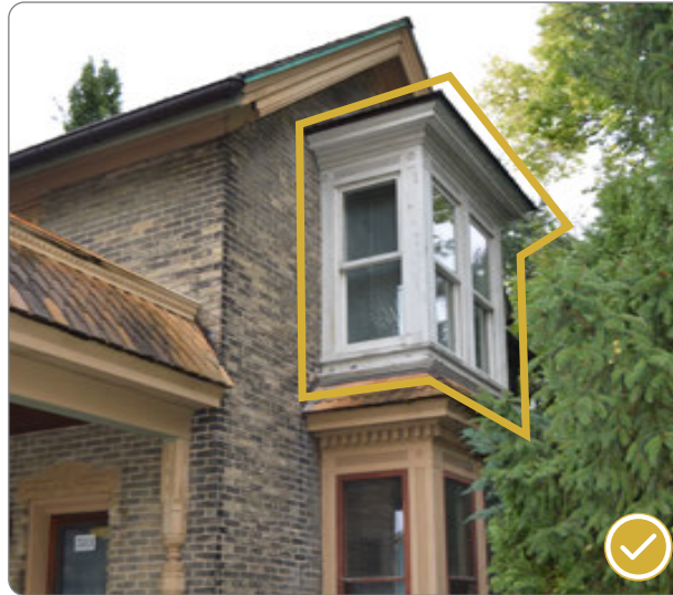
Figure 103: Compatible windows on a second story addition at 511 E Main Street (41.26.5.a-b).
