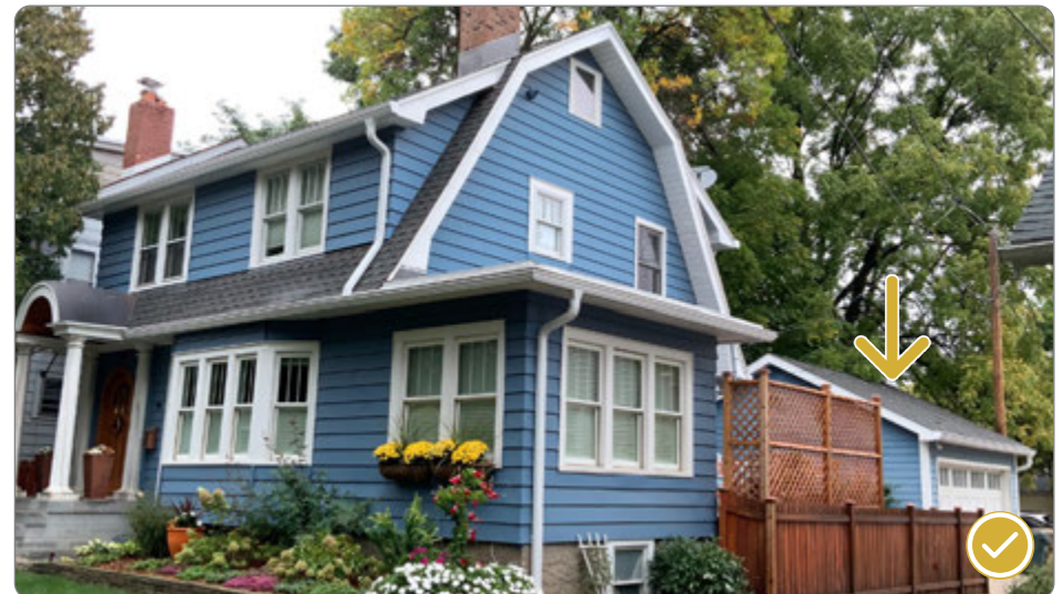
Figure 126: Compatible accessory structure at 905 Oakland Avenue (41.27.1.b).
