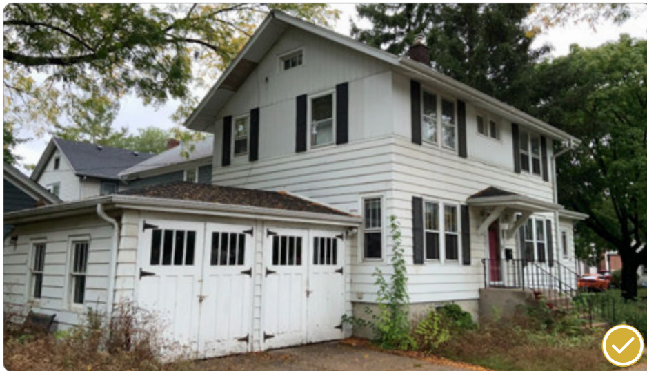
Figure 94: Compatible side addition on a residential building at 1608 Adams Street (41.26.3.a.1).
