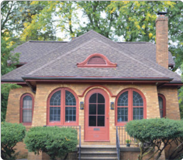
Figure 8: High Integrity Building - 624 S Thornton Avenue.
