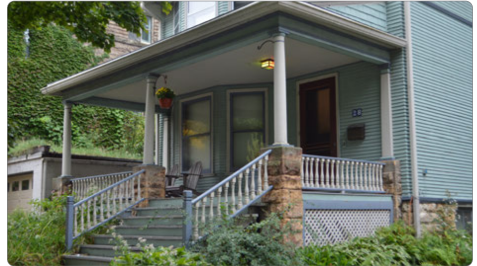
Figure 137: Porch details seen in Madison (41.27.6.a.1).
