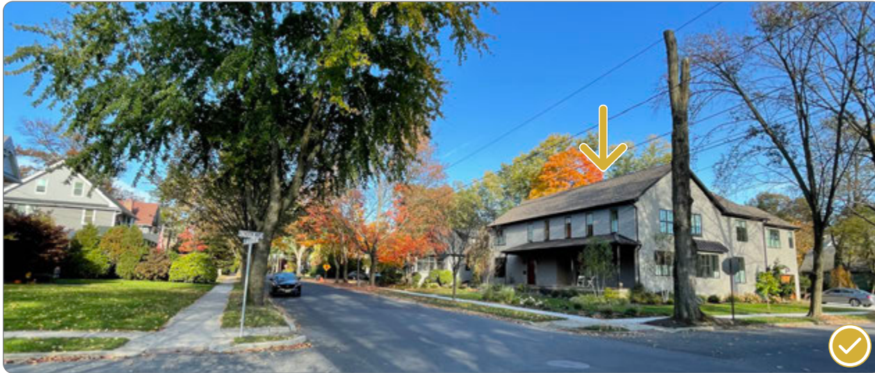
Figure 129: Infill construction demonstrating compatible wall material (41.27.3.a.1).
