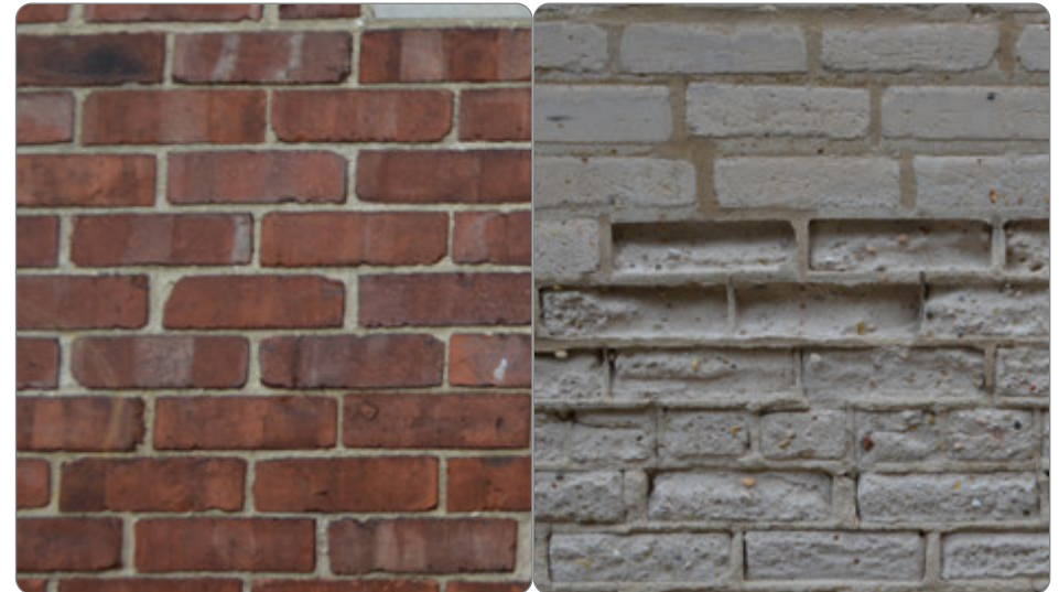
Figure 38: Proper vs. improper mortar alterations (41.24.2.a.1).
