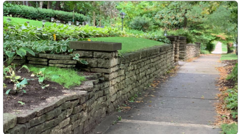
Figure 36: Retaining walls are considered a site feature (41.24.1.a.1).
