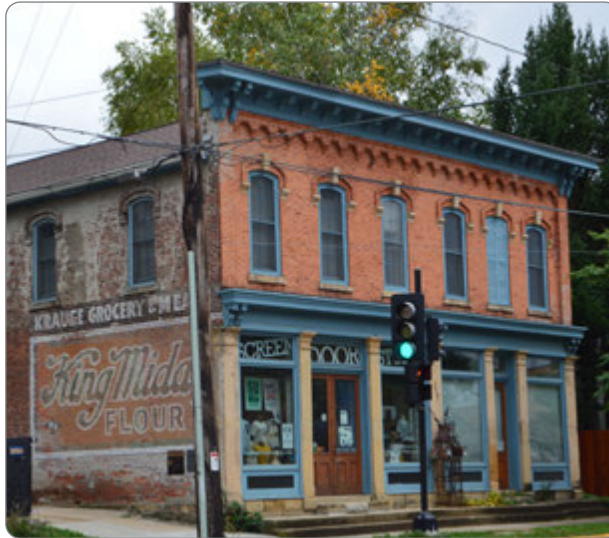
Figure 9: High Integrity Building - 853 Williamson Street.
