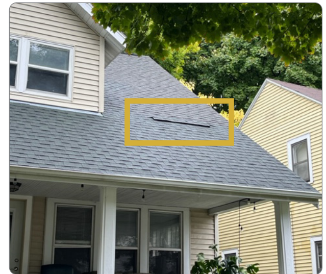
Figure 99: Minimally visible roof vent (41.26.4.e.1).
