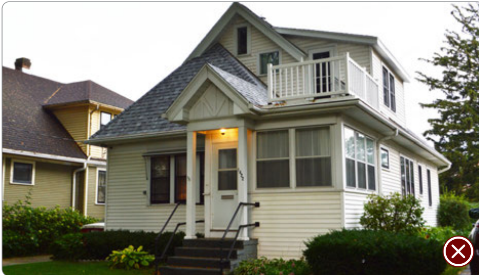
Figure 138: Incompatible front balcony addition (41.27.6.b.1).
