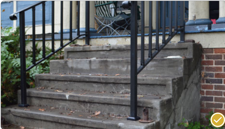
Figure 56: Compatible substitute metal railing replacement (41.25.3.c.1).
