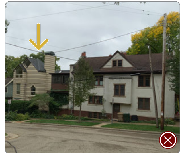
Figure 131: Infill construction demonstrating incompatible wall material (41.27.3.a.1).
