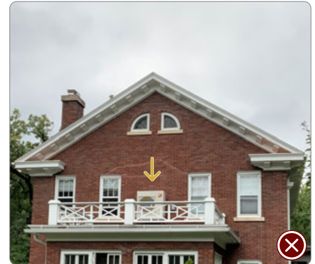
Figure 116: Mechanical equipment on front elevation of residence (41.26.7.1.2).
