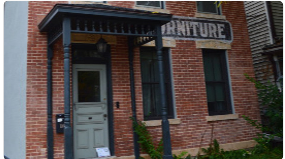
Figure 74: Example of a historically accurate entrance (41.25. 6).
