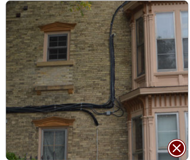
Figure 120: Exterior mounted conduit on historic building elevation (41.26.7.c.3).
