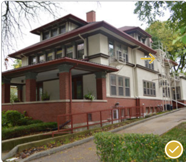
Figure 108: Example of a second exit stairway at 120 W Gorham Street (41.26.6.a.4).
