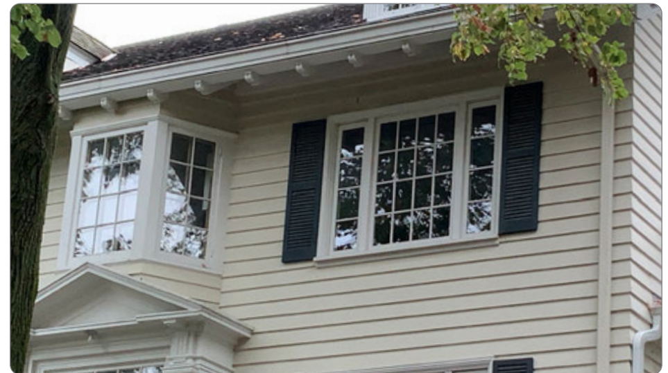
Figure 66: Replaced divided light windows (41.25.5.c.3).
