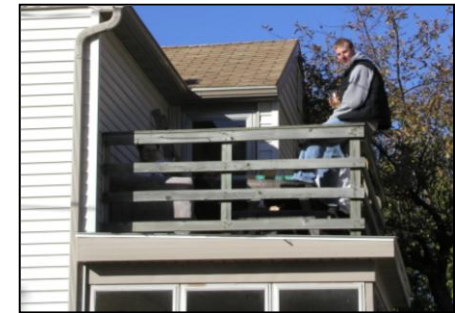
Decks throughout the neighborhood provide a diverse set of interactions and activities for neighborhood residents and visitors.
